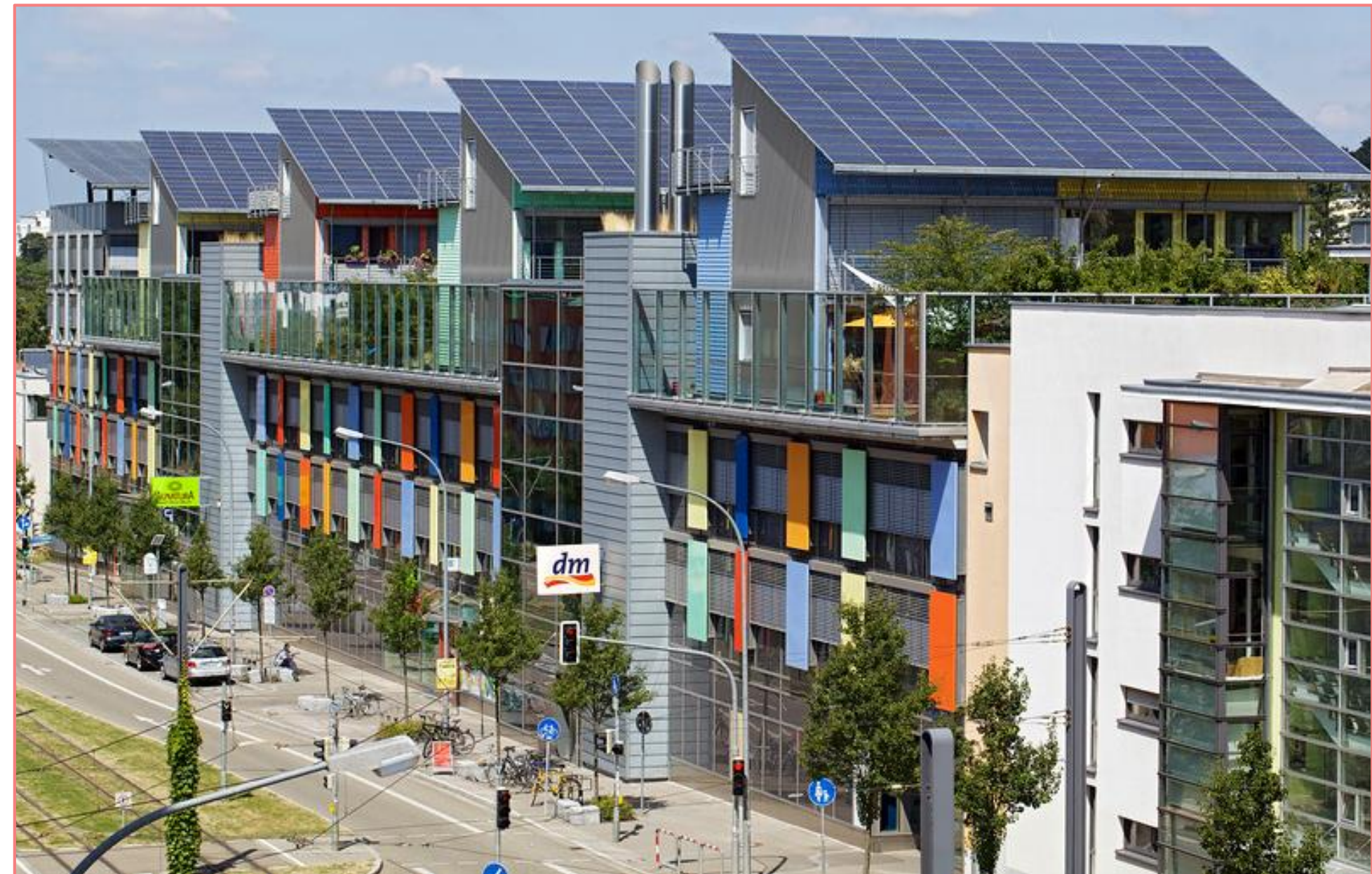
Example rooftops oriented to maximize solar access
