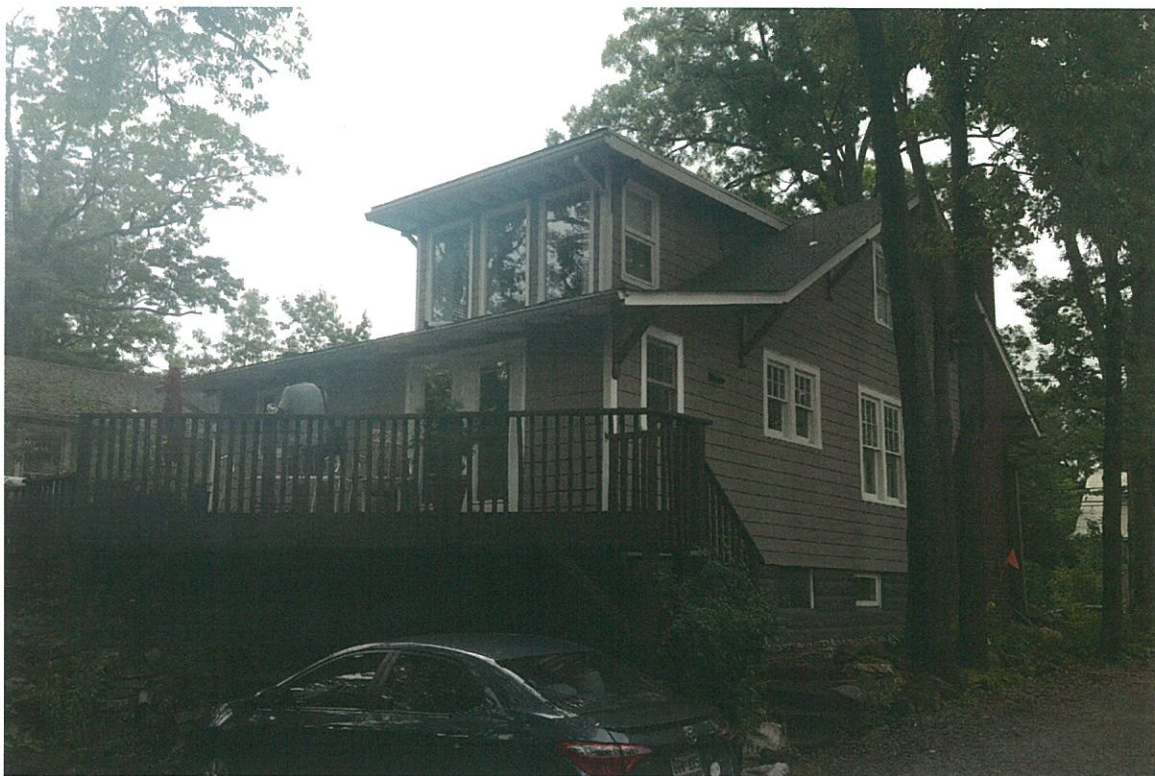
VIEW OF REAR OF EXIST. HOUSE
