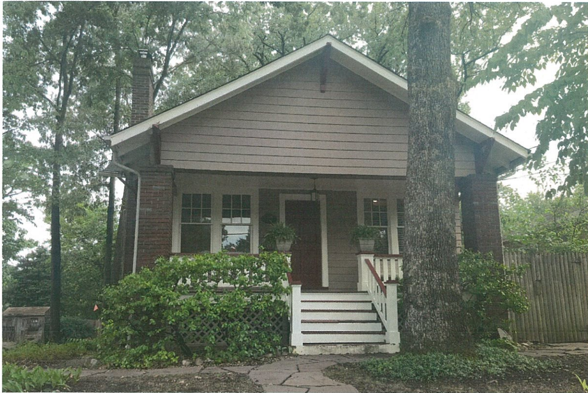
VIEW FROM STREET - FRONT OF EXIST. HOUSE
