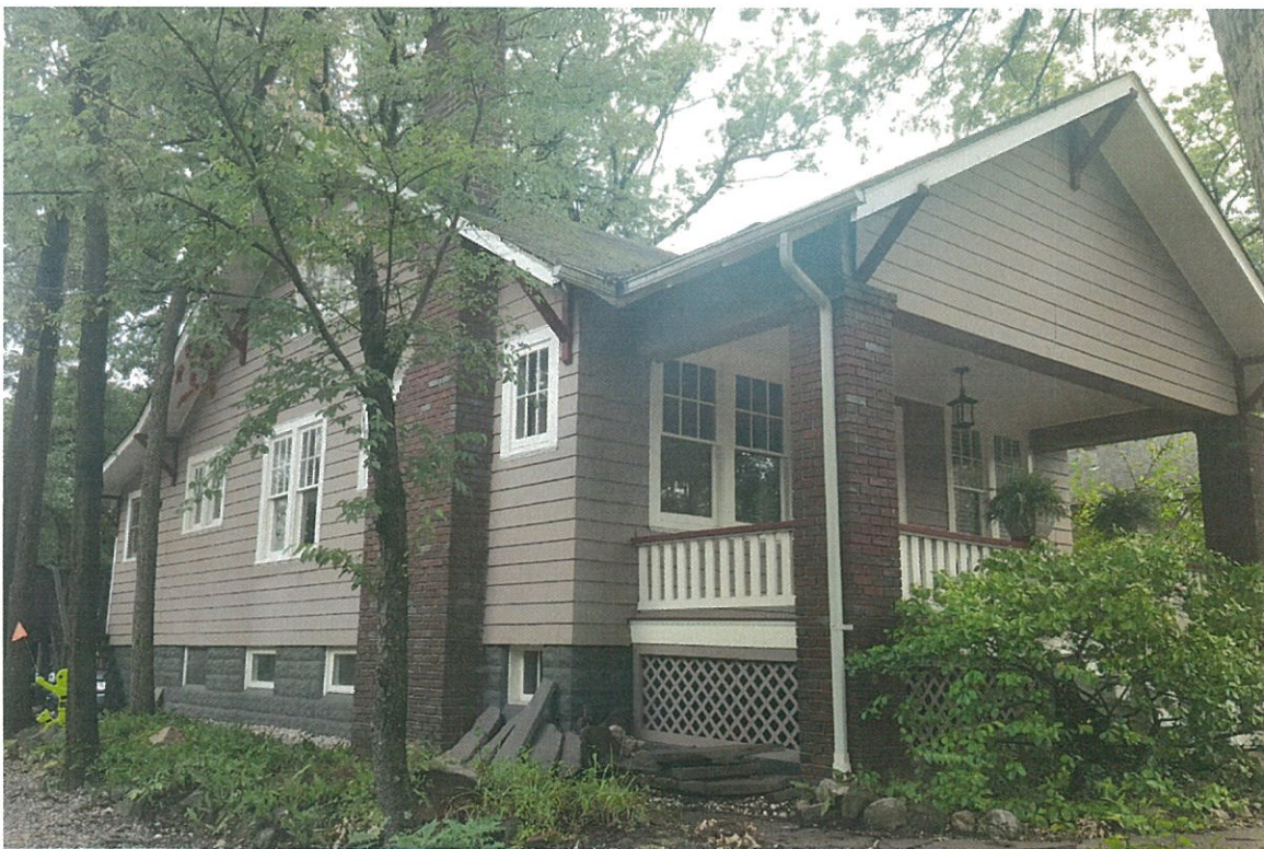
VIEW OF FRONT/EAST SIDE OF HOUSE
