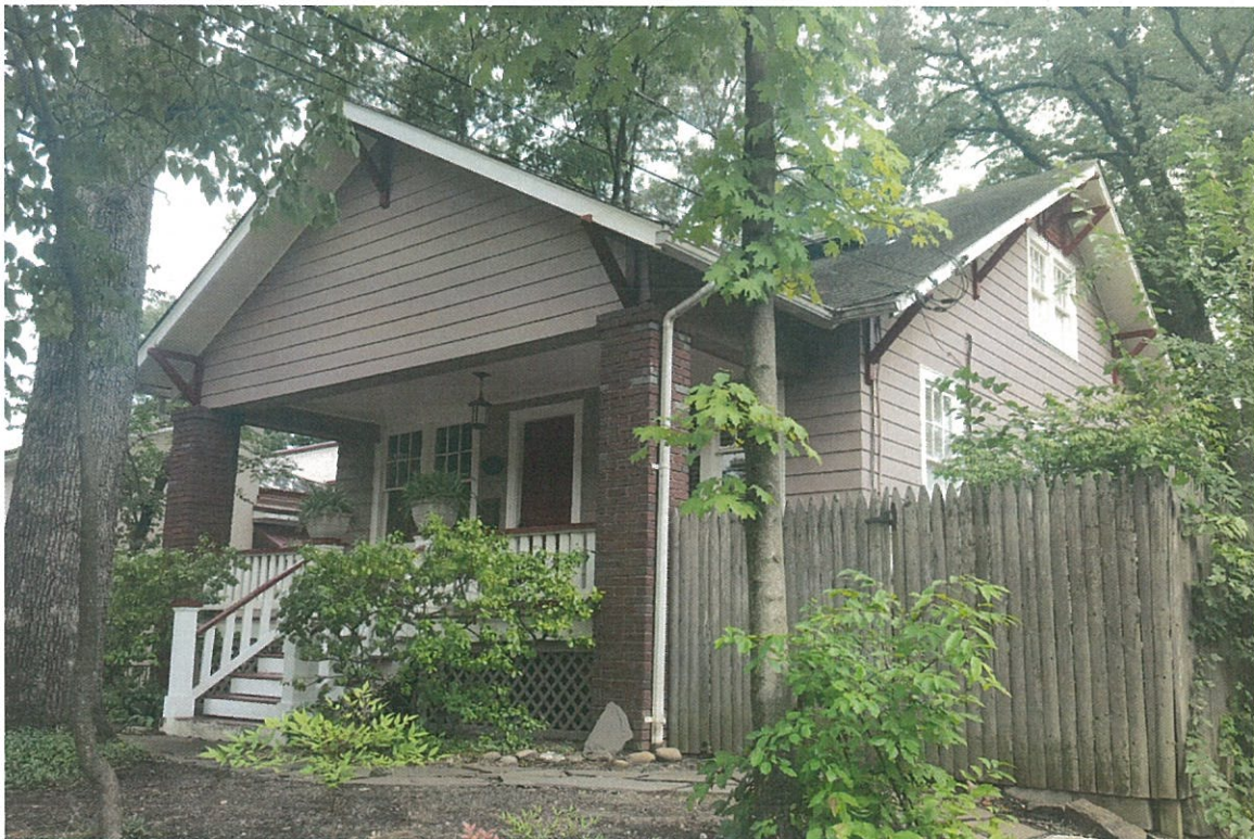
VIEW FROM STREET - FRONT/WEST VIEW OF HOUSE
