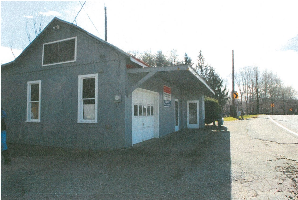
Figure 4 Existing front (west) facade with awning. Garage door to be replaced.
