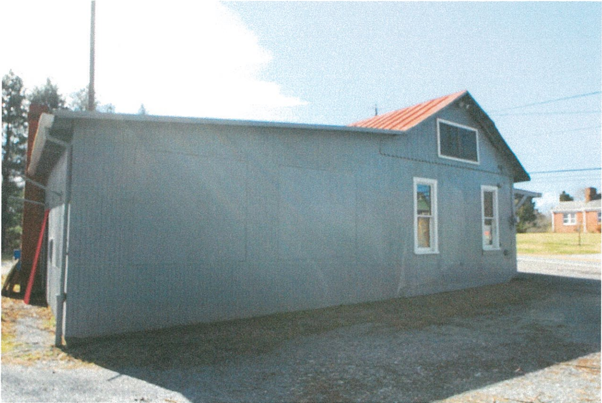
Figure 1 Existing North facade. Gable window will be removed and double hung windows will be replaced.
