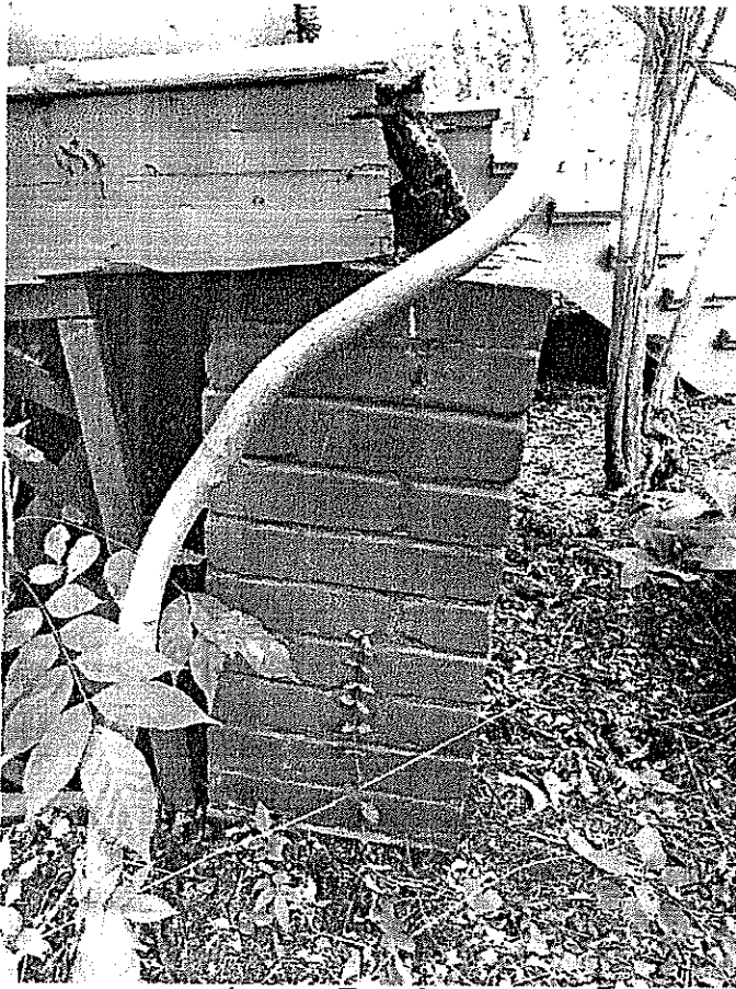
DETAIL: BRICK PIER @ LEFT SIDE
