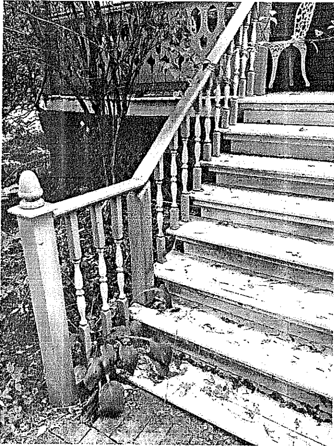
WOOD STAIR @ SIDE PORCH
