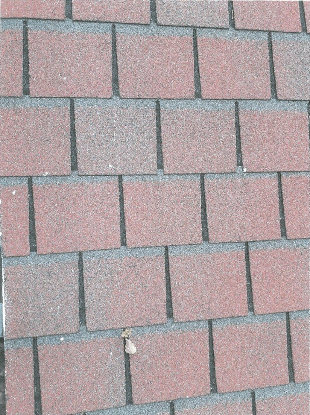
Good shingles on South Side of Barn (Certainteed, Discontinued)
