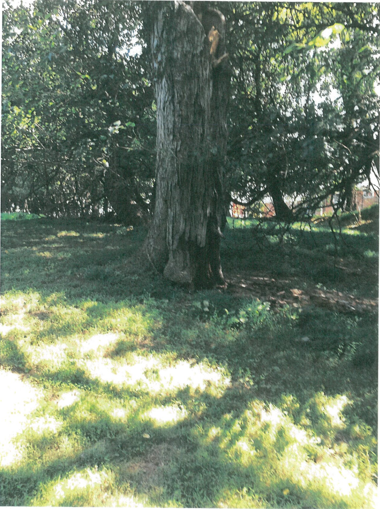
Detail: Severe trunk and internal tree decay
