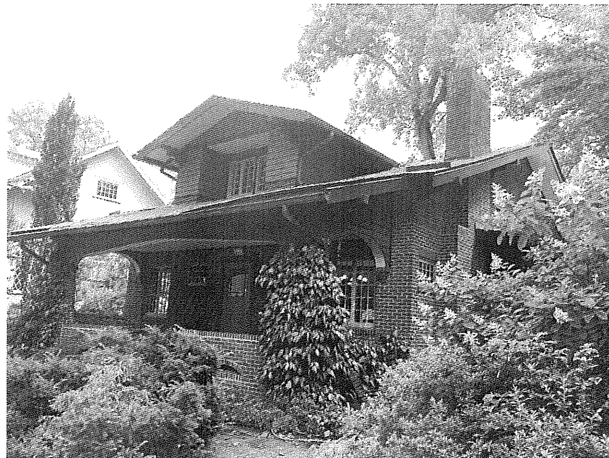
FRONT (VIEWED FROM WEST KIRKE STREET)
