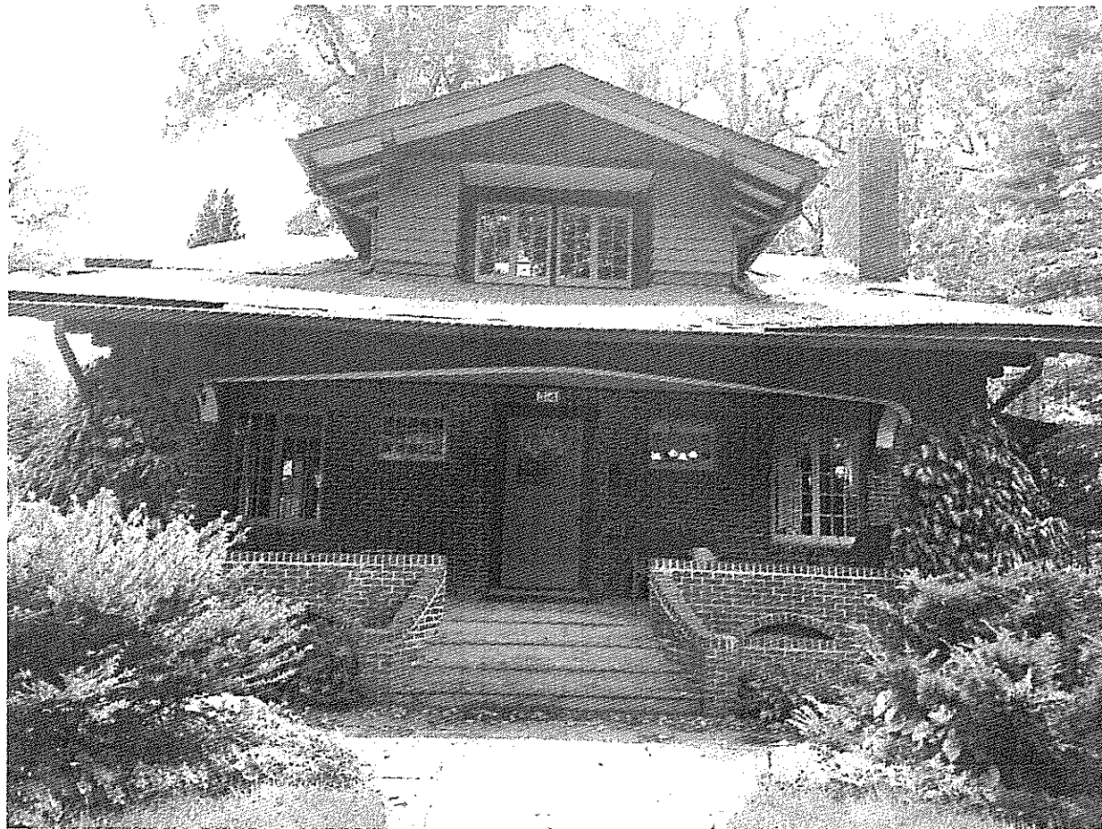
FRONT (VIEWED FROM WEST KIRKE STREET)
