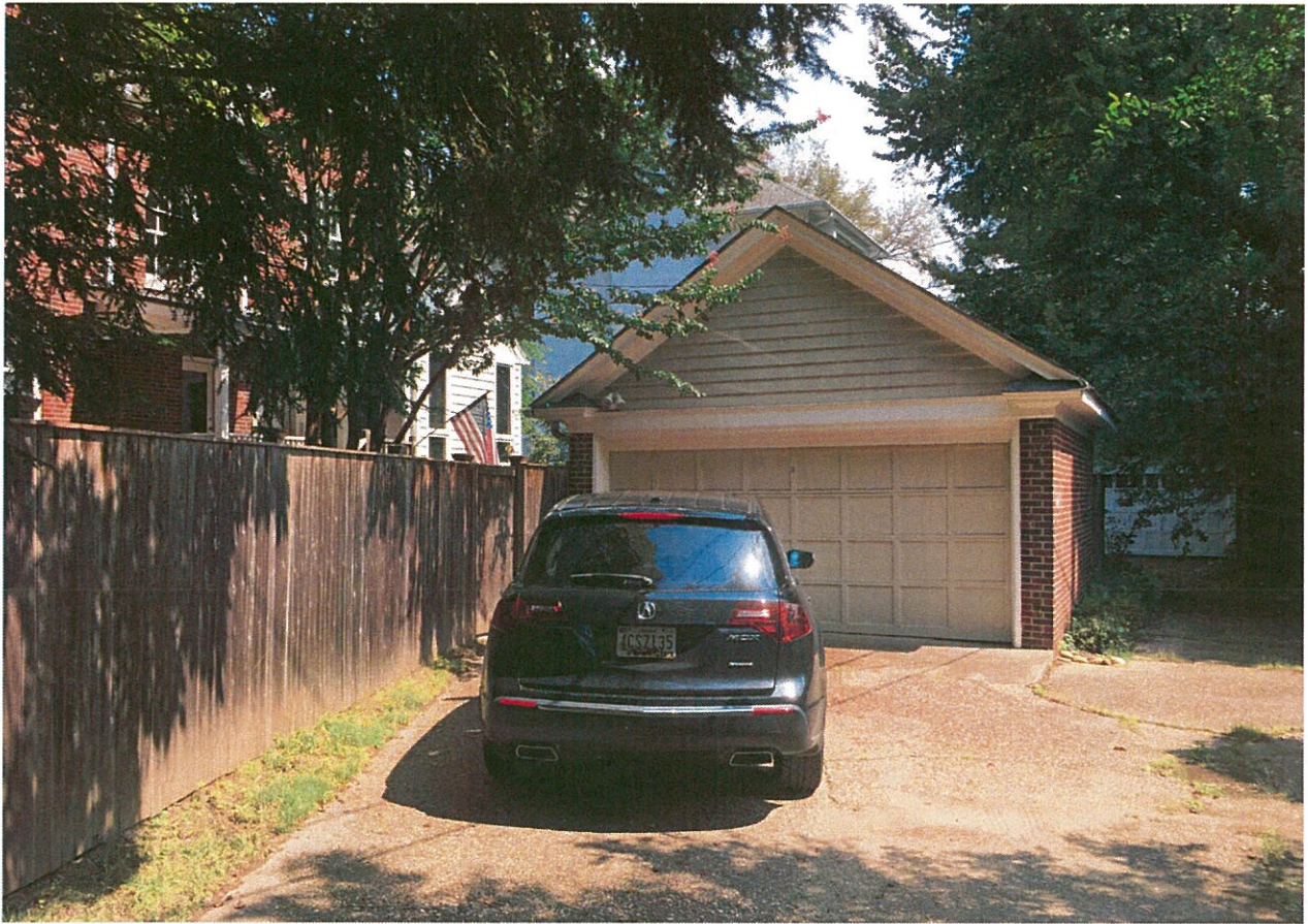
▲ ABOVE: VIEW OF EXISTING GARAGE (NO WORK) AND PARTIAL VIEW OF EXISTING ADDITION TO BE DEMOLISHED (WHITE SIDING)
