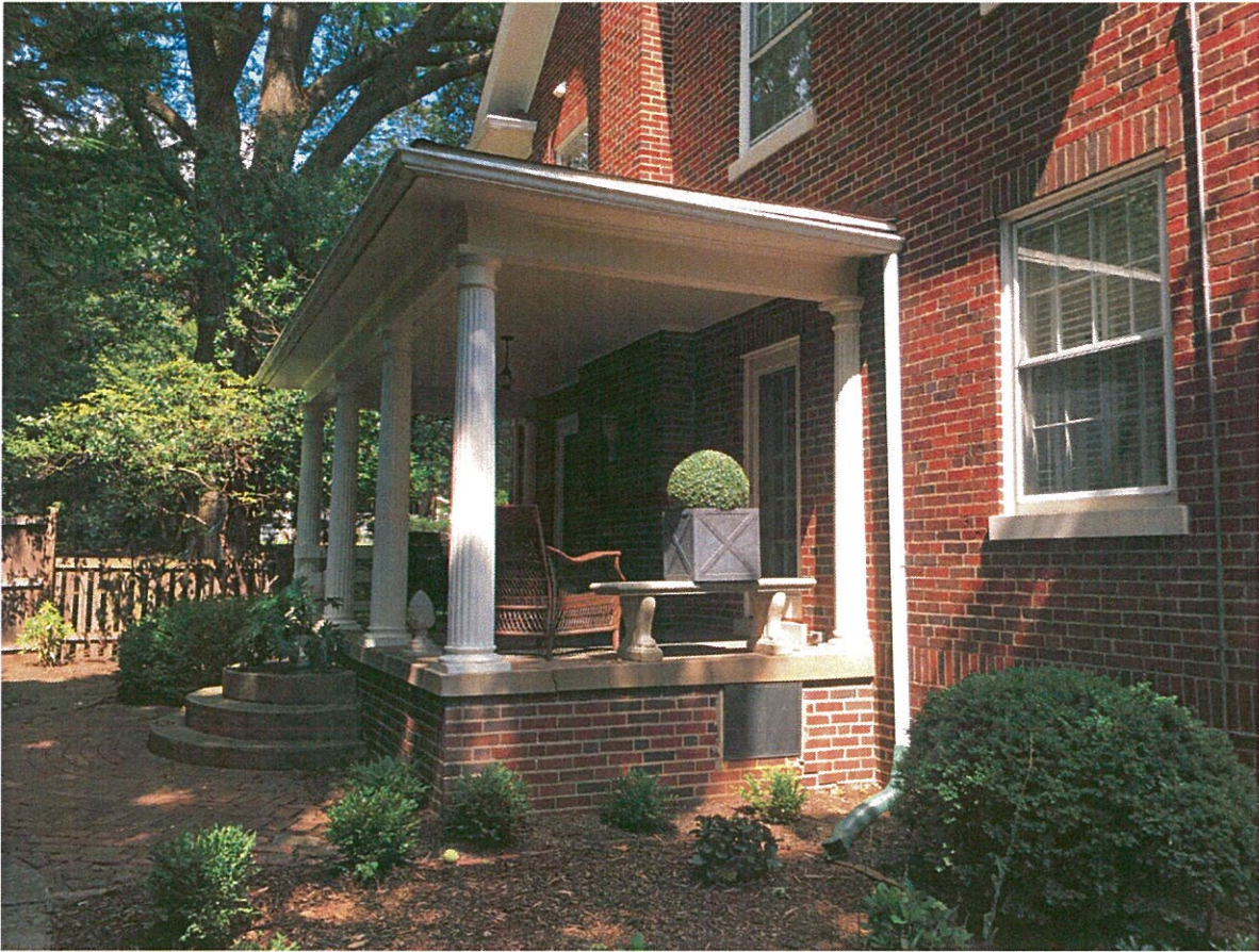
A ABOVE: CONTEXTUAL VIEW OF EXISTING RIGHT SIDE OF HOUSE AND COVERED PORCH. NO WORK PROPOSED.
