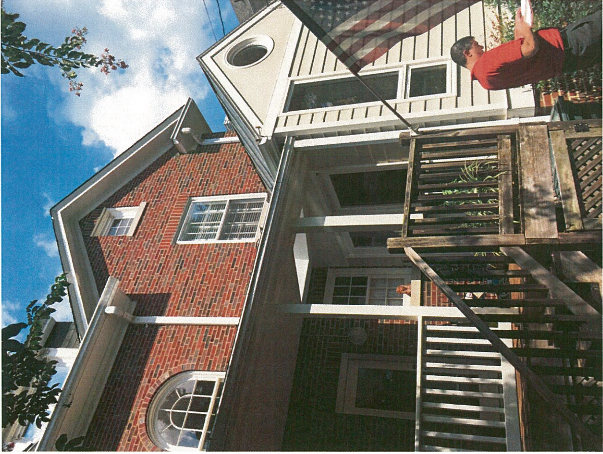
VIEW OF EXISTING ADDITION AND COVERED PORCH AT REAR OF HOUSE TO BE DEMOLISHED FOR NEW ADDITION.
