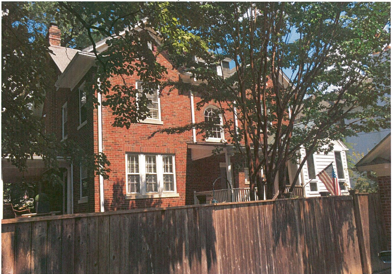
▼ BELOW: VIEW OF EXISTING REAR ELEVATION WITH COVERED PORCH AND EXISTING ADDITION (STRUCTURE WITH WHITE SIDING), BOTH STRUCTURES TO BE DEMOLISHED FOR NEW ADDITION.
