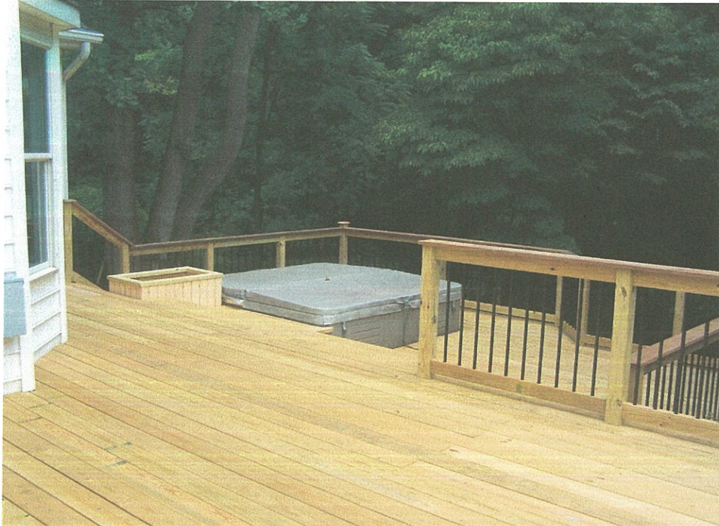
Sample Railing: #1 grade Pressure Treated Pine with Black Aluminum Balusters and Ipe Cap.
