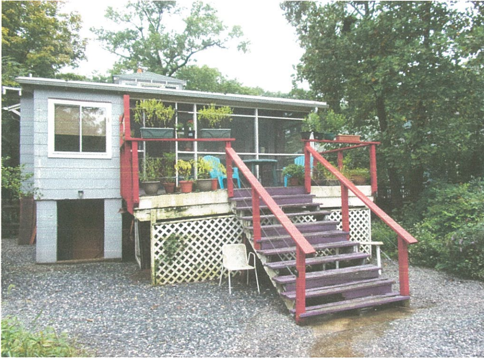
Existing porch and deck is unsafe and not to present building code.
