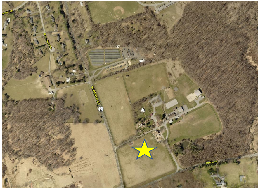
Figure 1: Woodlawn is a collection of early 19 th century buildings.
