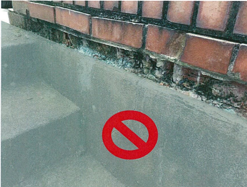
Detail: Current driveway / basement wall.
