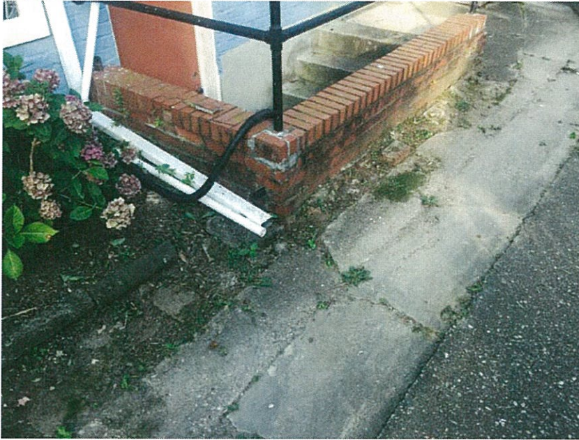
Detail: Current driveway / basement wall.
