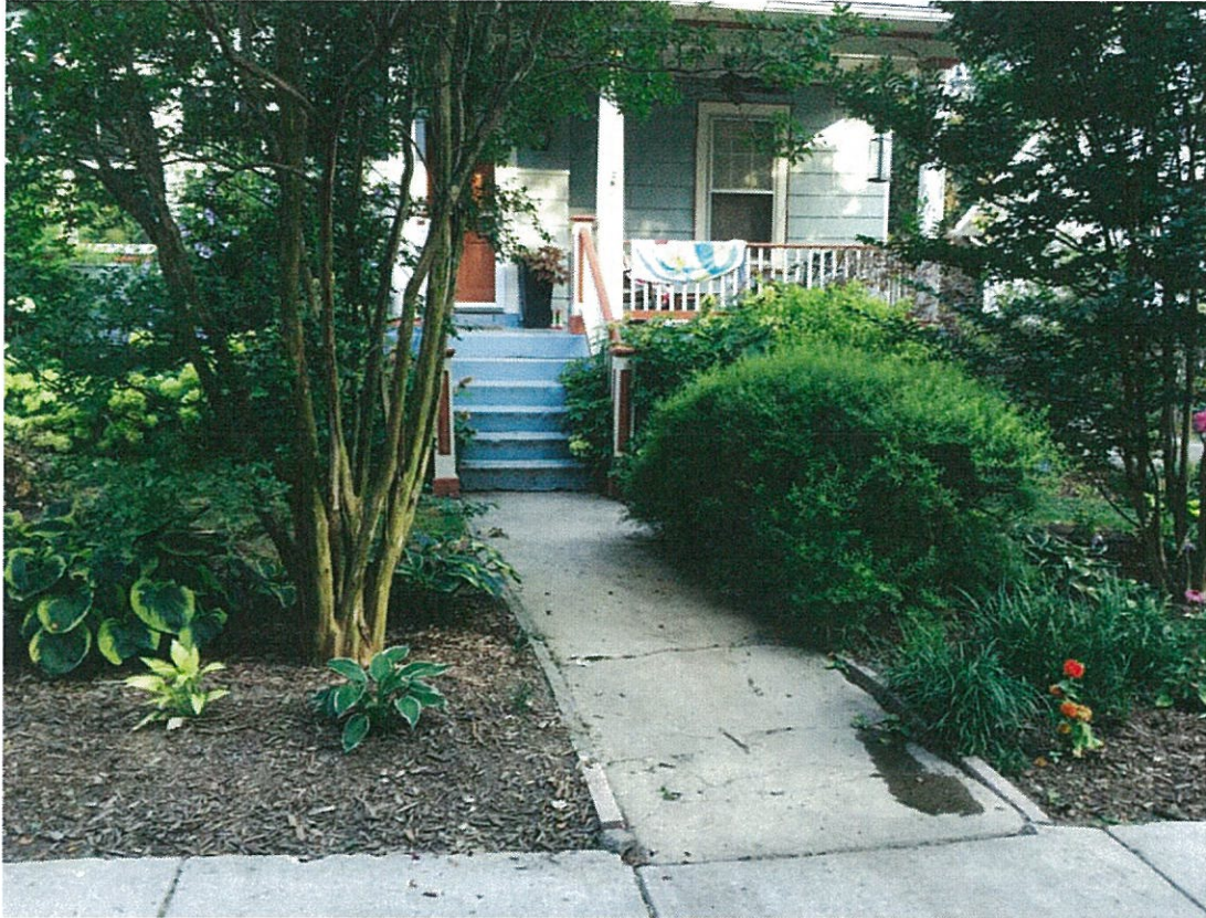
Detail: Current poured concrete walkway in front yard.
