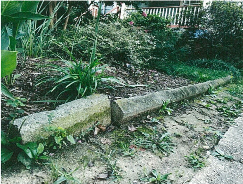
Detail: Current driveway concrete block curb.
