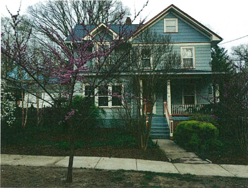
Detail: Front of 7204 Spruce Ave., Takoma Park, Maryland.
