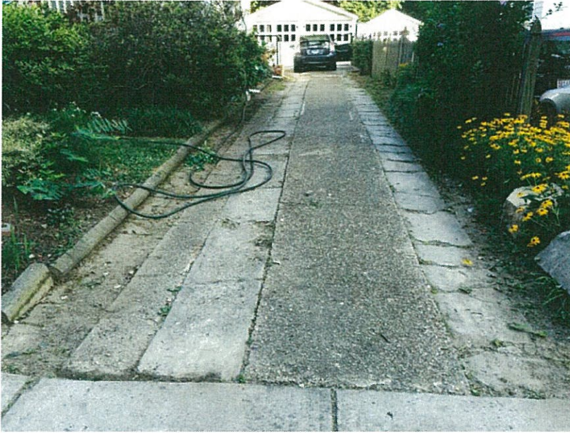
Detail: Current driveway concrete block curb.
