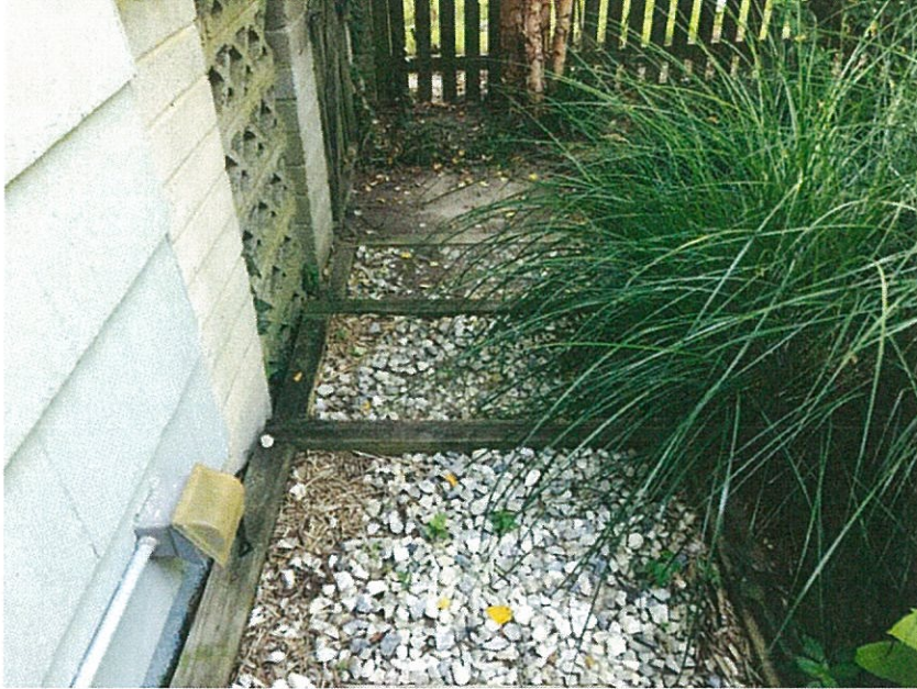
Detail: Current rear left loose stone and pressure-treated timber walkway in back yard.
