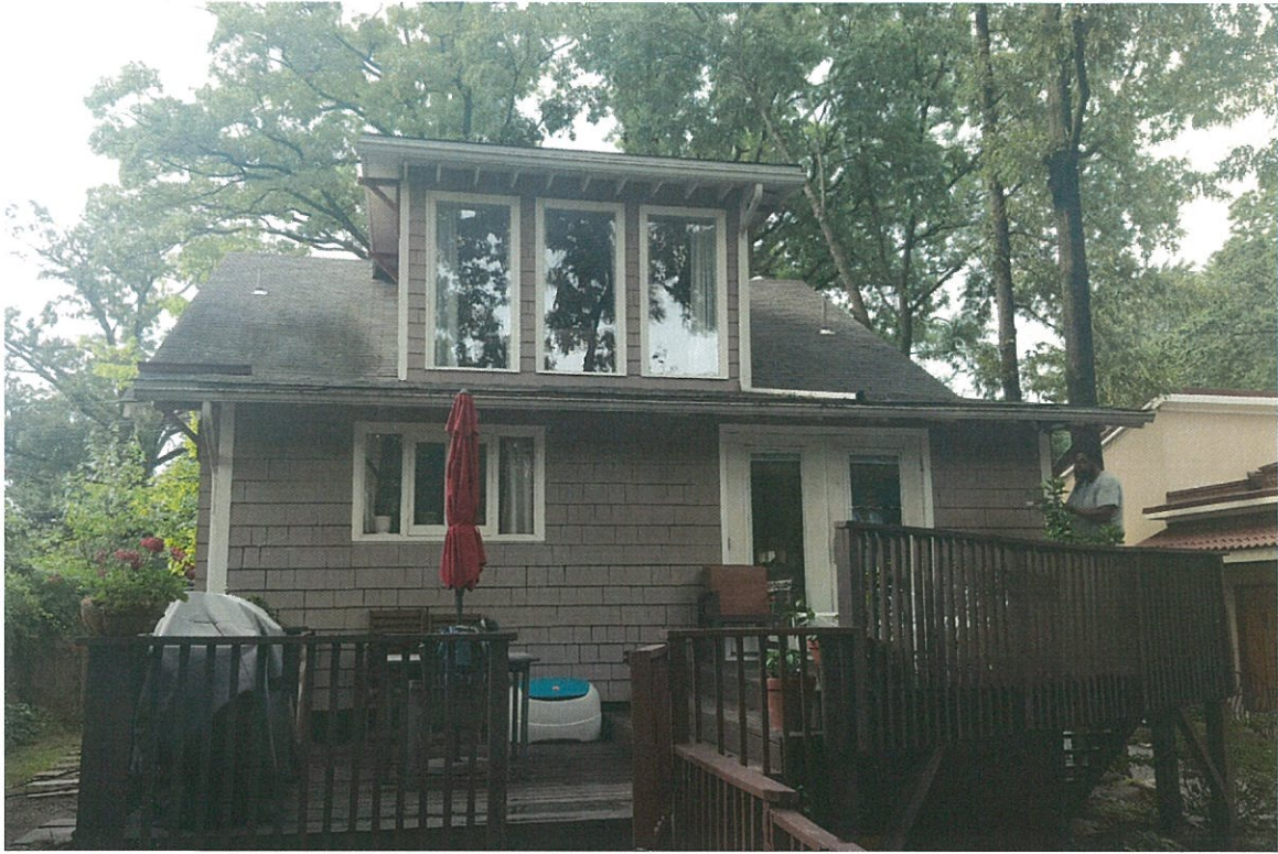
VIEW OF REAR OF EXIST. HOUSE
