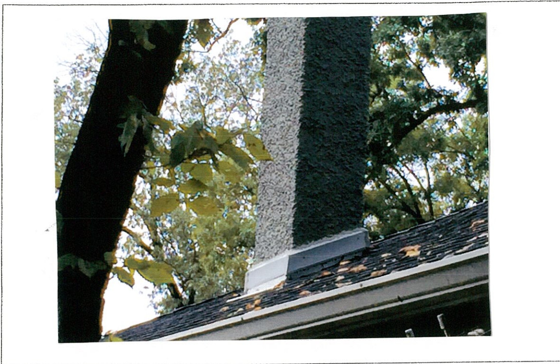
Detail: close-up of our 2 nd chimney
