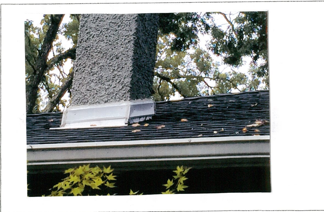
Detail: Close-up of unconnected + unused chimney in the walls of our house
