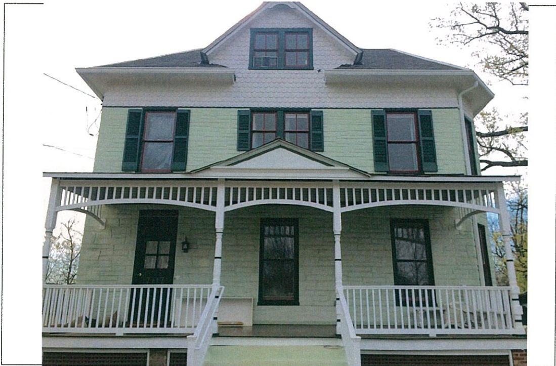
Detail: Front facade
