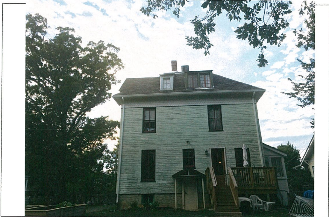
Detail: Rear facade
