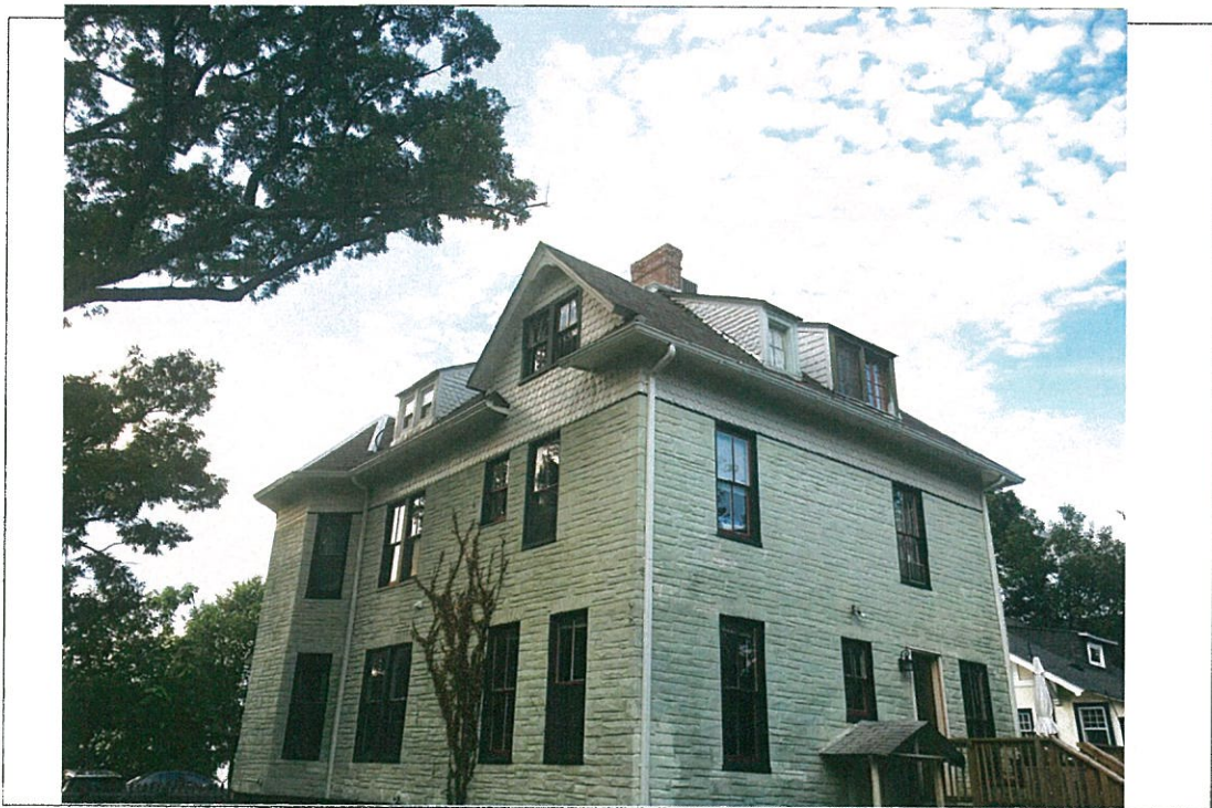
Detail: South (side) facade
