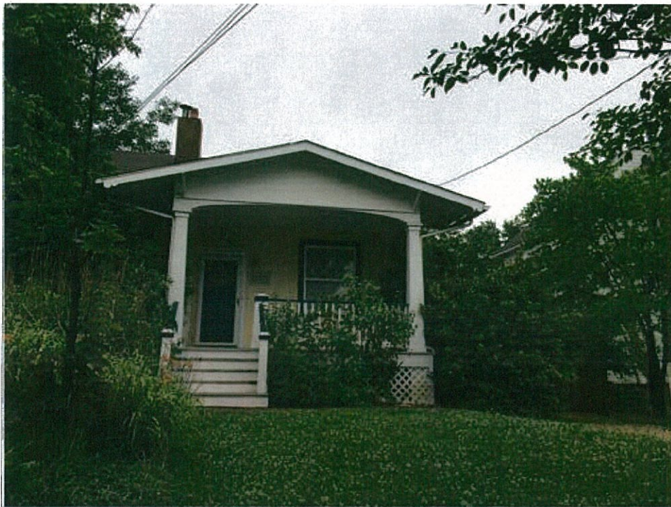
Detail: North adjacent neighbor from public right of way 7121 Carroll
