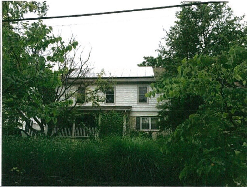
Detail: South rear-adjacent neighbor from public right of way 26 Columbia
