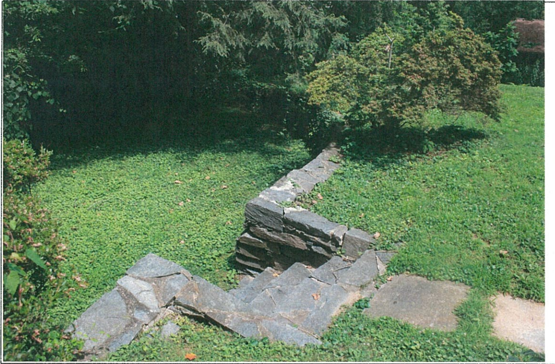
Detail: ORIGINAL SIDE YARD RETAINING WALL
