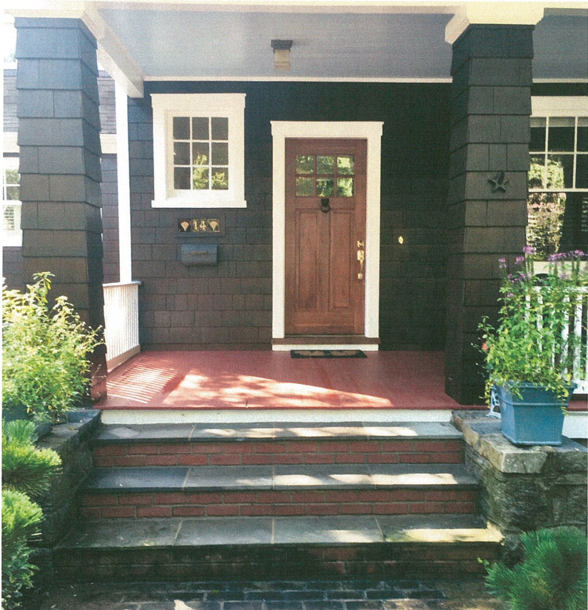
Existing front stairs without railings.
