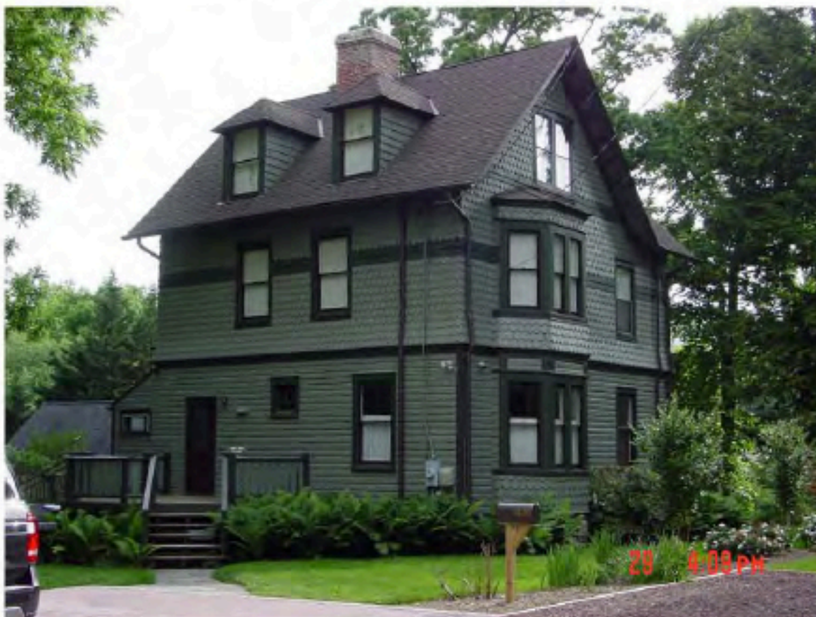
Detail: Rear and Partial North Elevations from Lee St. ROW
