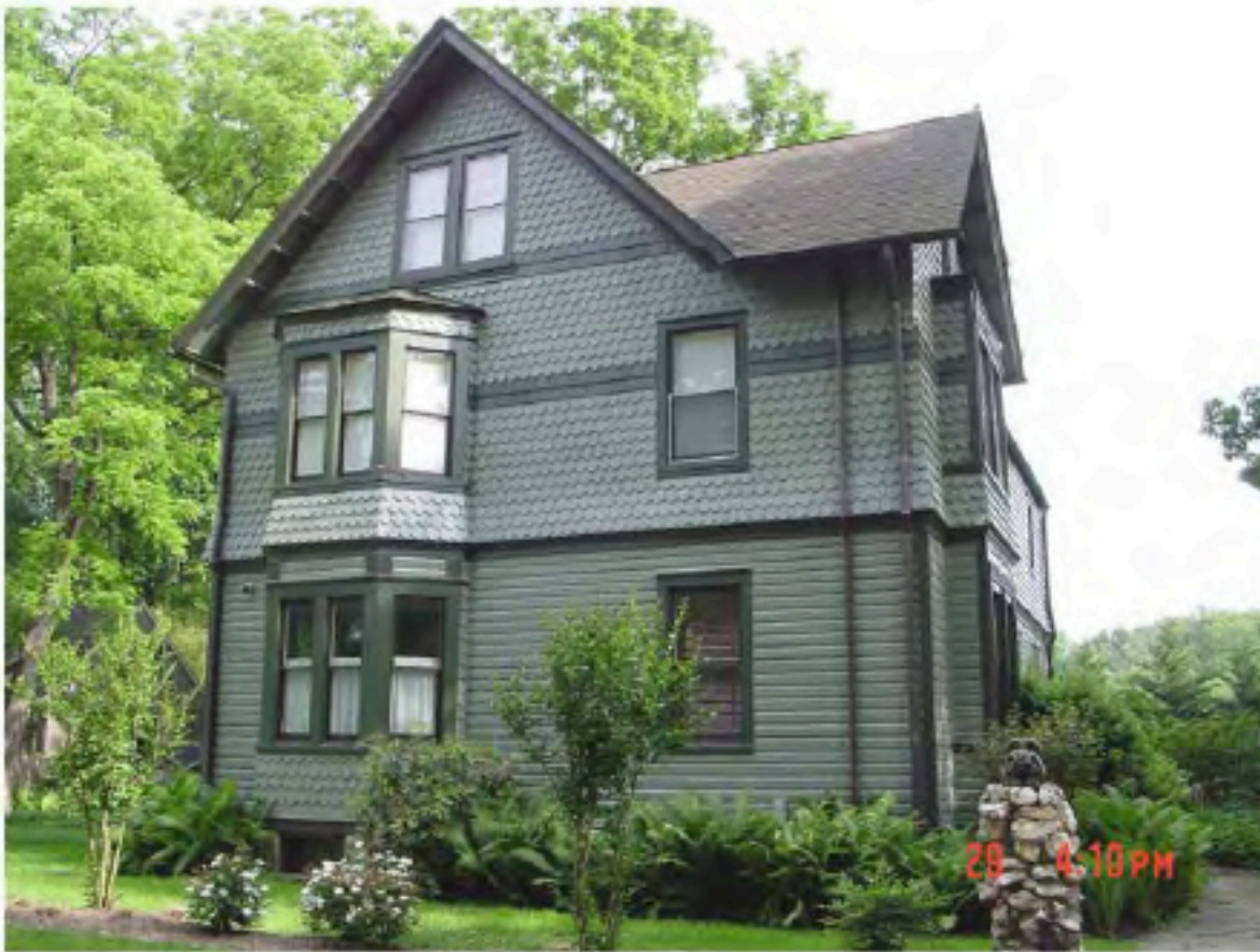
Detail: North Elevation from Lee St. ROW
