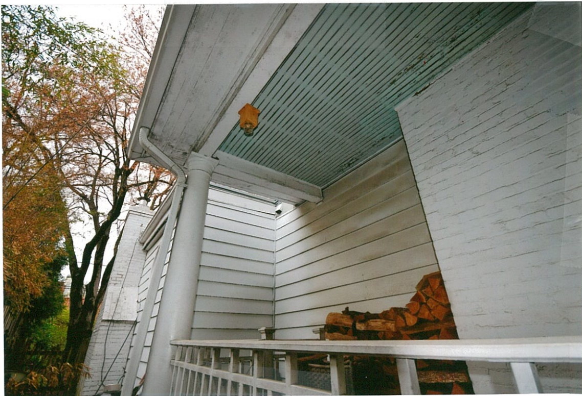
Detail Photo#34 4/25/18 Side (west) elevation showing rear side of wraparound porch, aluminum siding to be removed, woodwork needing painting
