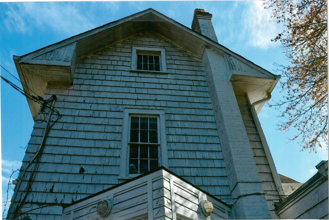
Detail Photo#24 4/25/18 Rear (north) elevation showing 3-story oldest part of house with original cedar shingles needing paint, plus top vee-shaped kitchen bay
