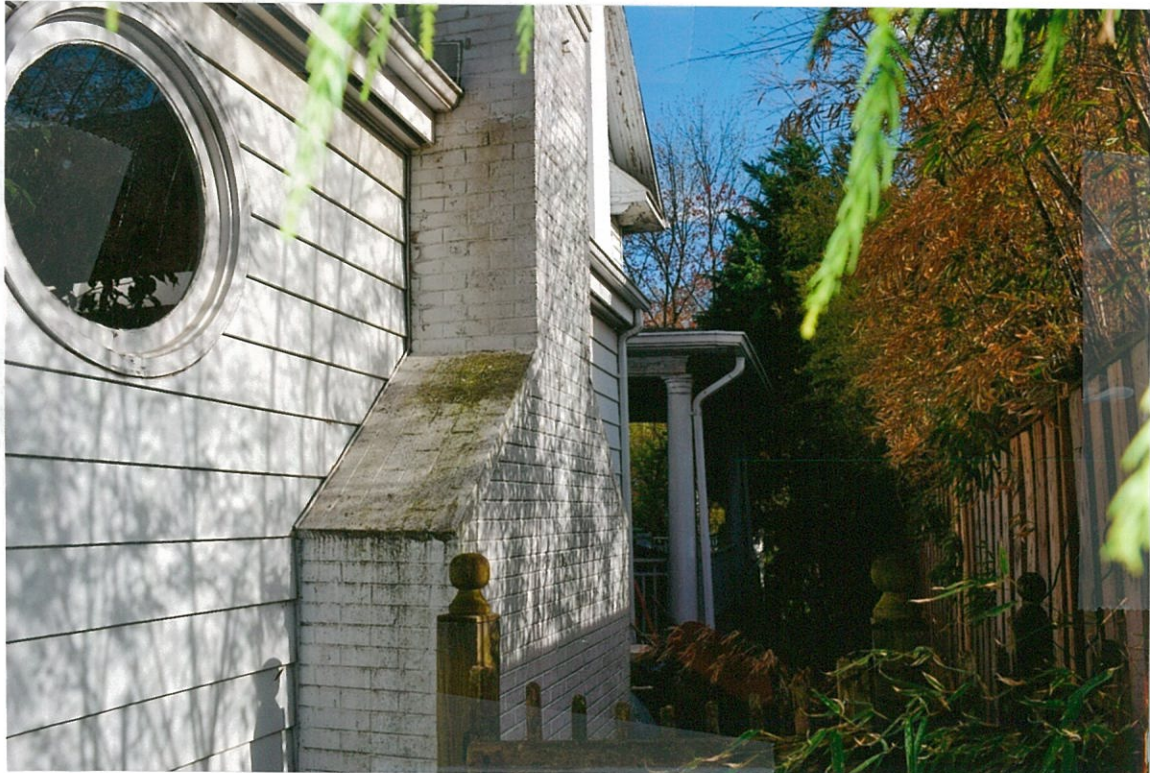
Detail Photo#36 4/25/18 Side (west) elevation showing exterior of family room, aluminum siding to be removed, woodwork needing painting
