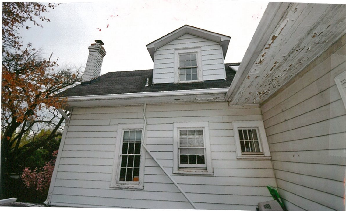
Detail Photo# 39 40 4/25/18 rear (north) elevation and side (west) elevation showing 2 nd floor exterior and family room roof, aluminum siding to be removed, eaves and woodwork needing painting
