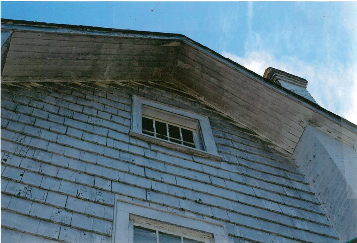
Detail Photo#29 4/25/18 Side (east) elevation showing 3rd-floor window aluminum siding to be removed, eaves needing painting
