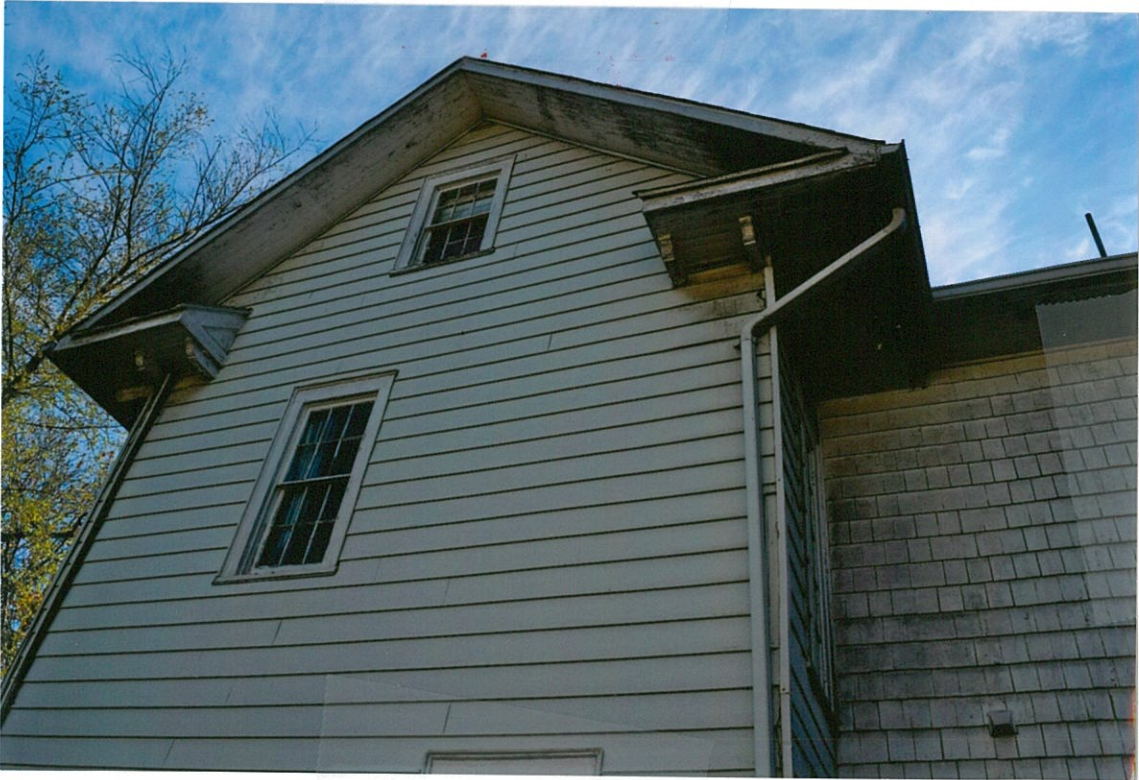
Detail Photo#28 4/25/18 Side (east) elevation showing aluminum siding to be removed, eaves needing painting
