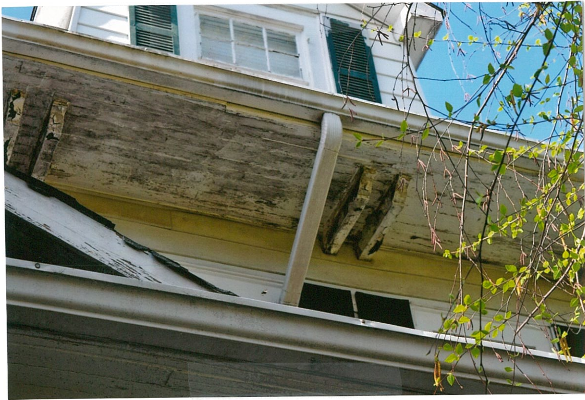
Detail Photo#19 4/25/18 Front (south) elevation Front (south) elevation, detail of eaves showing peeling paint and mildew
