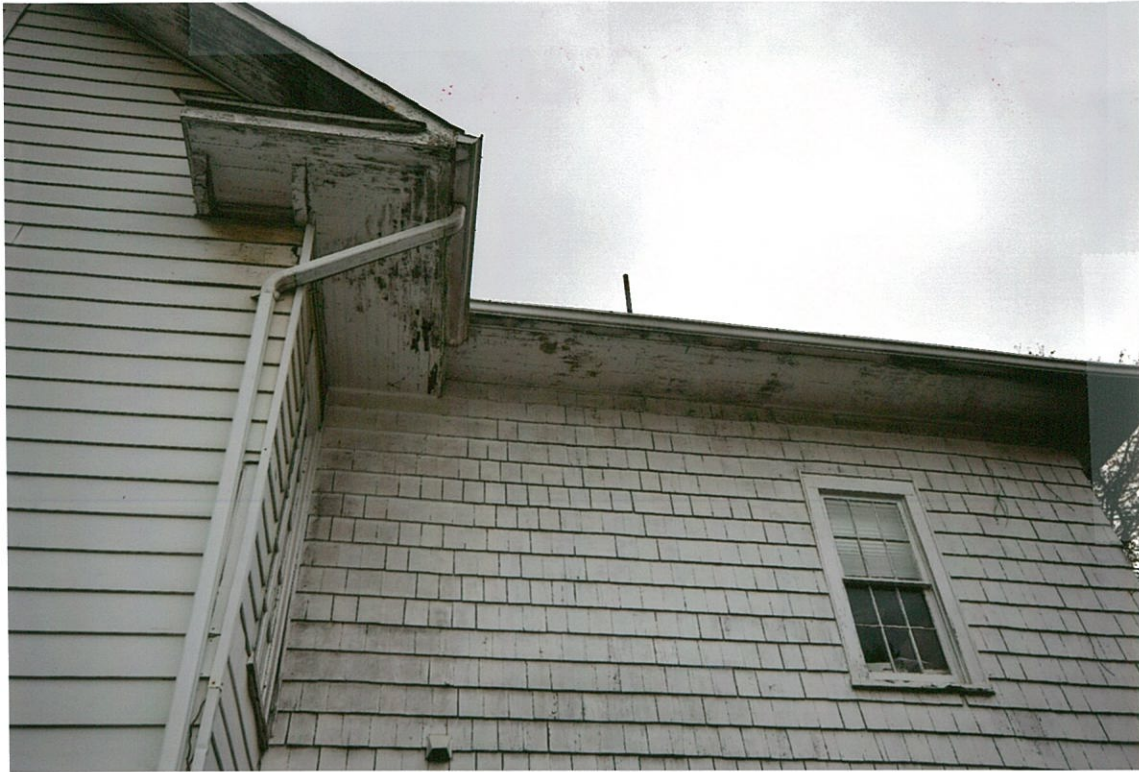
Detail Photo#31 4/25/18 Side (east) elevation showing 2 nd floor windows, original cedar siding, woodwork and eaves needing painting
