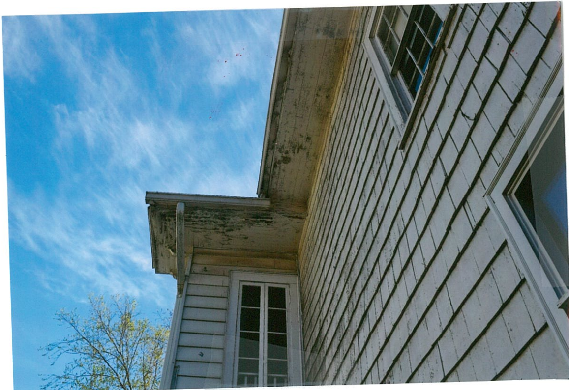
Detail Photo#32 4/25/18 Side (east) elevation showing 2 nd floor windows, original cedar siding, woodwork and eaves needing painting
