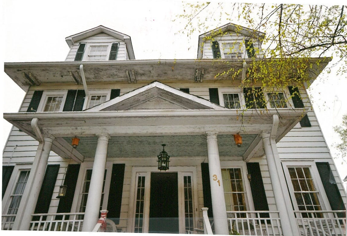
Detail Photo# 7 4/25/18 Front (south) elevation Shows mildew, peeling paint under eaves aluminum siding to be removed
