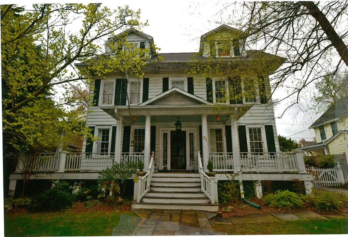
Detail: Photo# 1 4/25/18 Front (south) elevation
