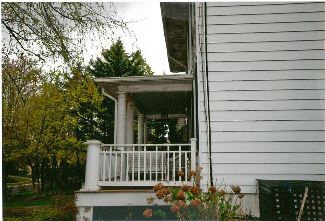
Detail Photo#18 4/25/18 side (east) elevation Side of front porch and beginning of east elevation, showing aluminum siding to be removed.
