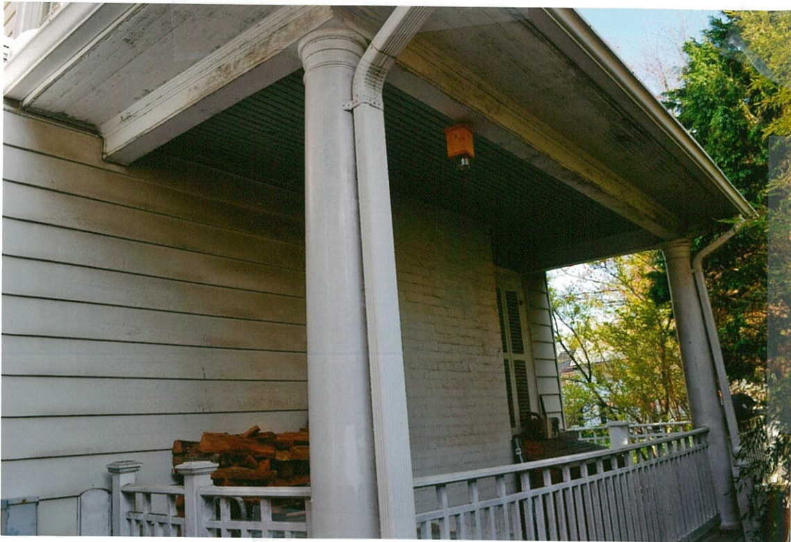
Detail Photo#33 4/25/18 Side (west) elevation showing rear side of wraparound porch, aluminum siding to be removed, woodwork needing painting
