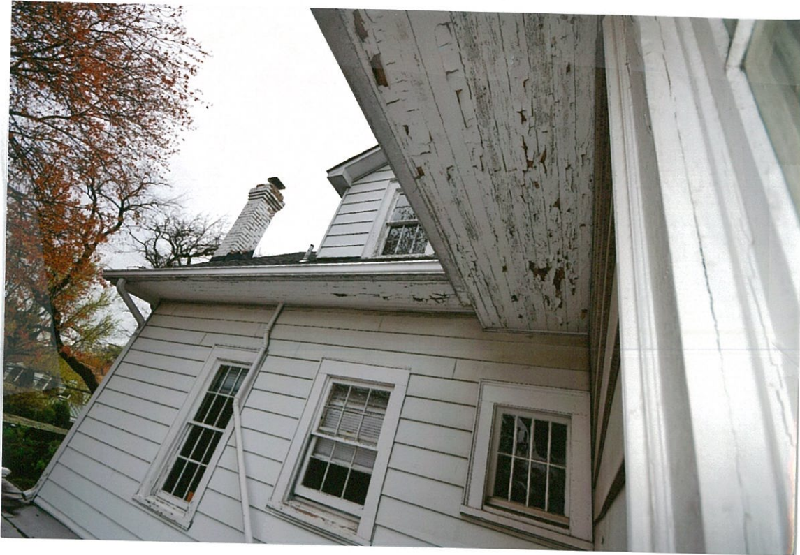
Detail Photo#39 4/25/18 rear (north) elevation and side (west) elevation showing 2 nd floor exterior and family room roof, aluminum siding to be removed, eaves and woodwork needing painting
