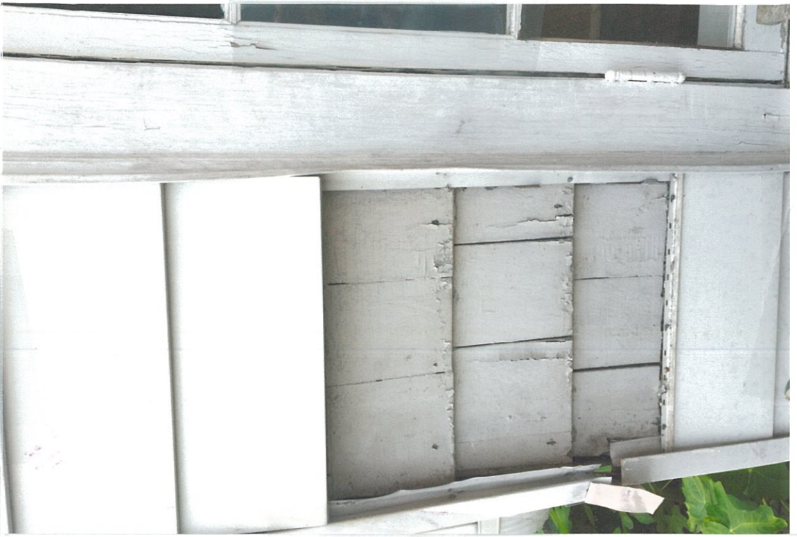
Detail Photo#45 8/22/18 side (east) elevation showing detail of aluminum siding to be removed and original cedar siding underneath
