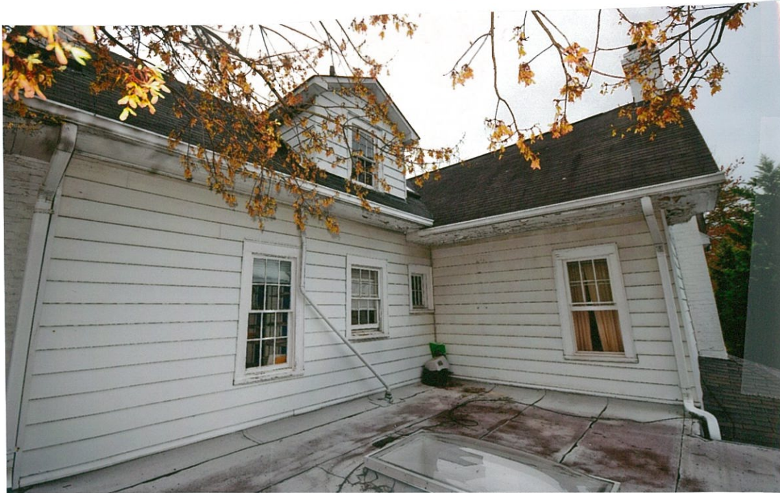
Detail Photo#38 4/25/18 rear (north) elevation and side (west) elevation showing 2 nd floor exterior and family room roof, aluminum siding to be removed, eaves and woodwork needing painting
