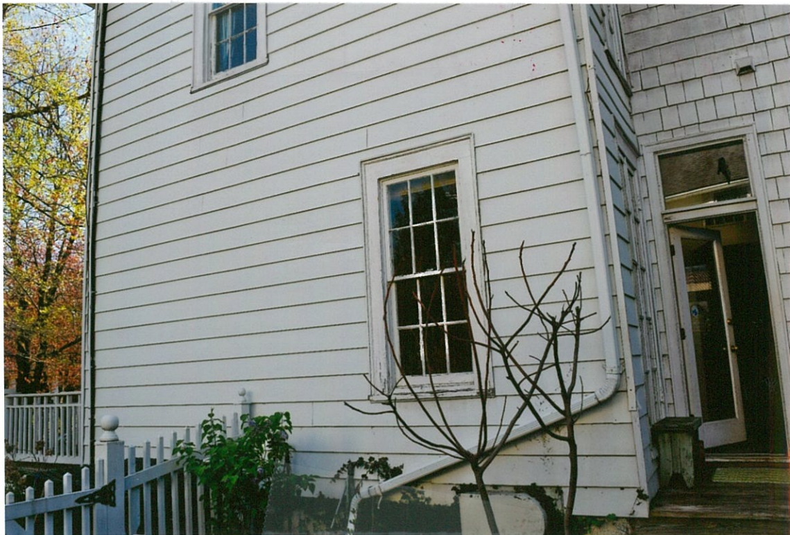
Detail Photo#26 4/25/18 Side (east) elevation showing 1 st -floor side door aluminum siding to be removed
