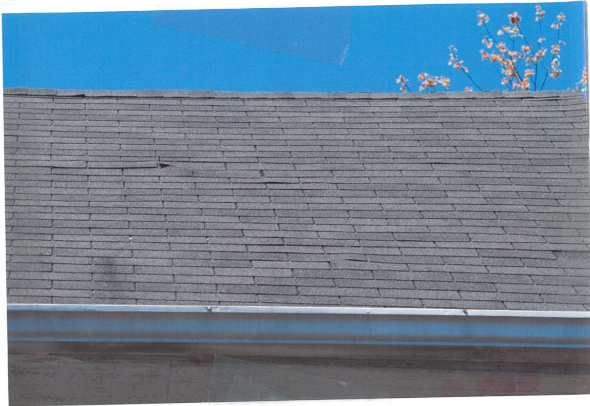
Detail Photo#43 rear (north) elevation roof showing missing and irregular shingles
