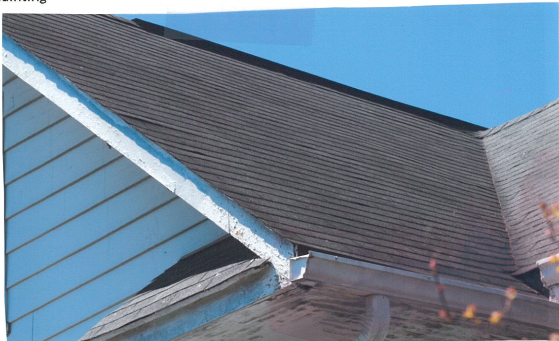
Detail Photo# 41 4/25/18 rear (north) elevation and side (west) elevation showing 2 nd floor exterior and family room roof, aluminum siding to be removed, eaves and woodwork needing painting
