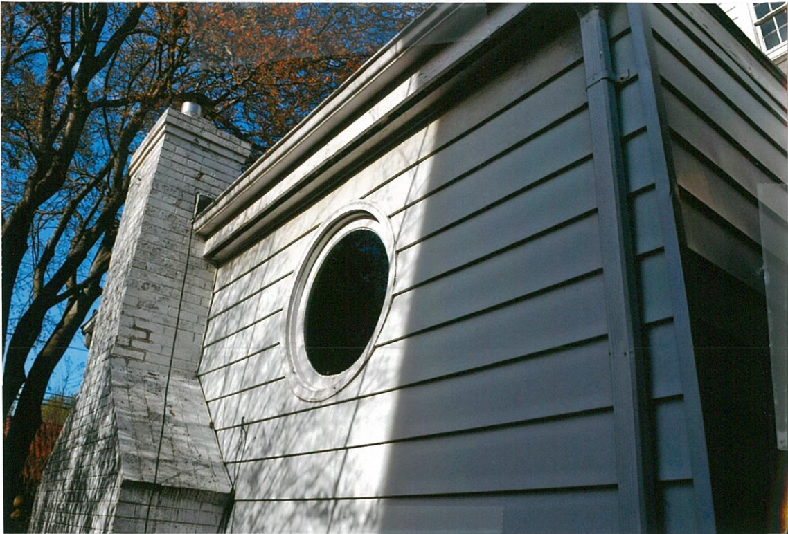
Detail Photo#35 4/25/18 Side (west) elevation showing exterior of family room, aluminum siding to be removed, woodwork needing painting
