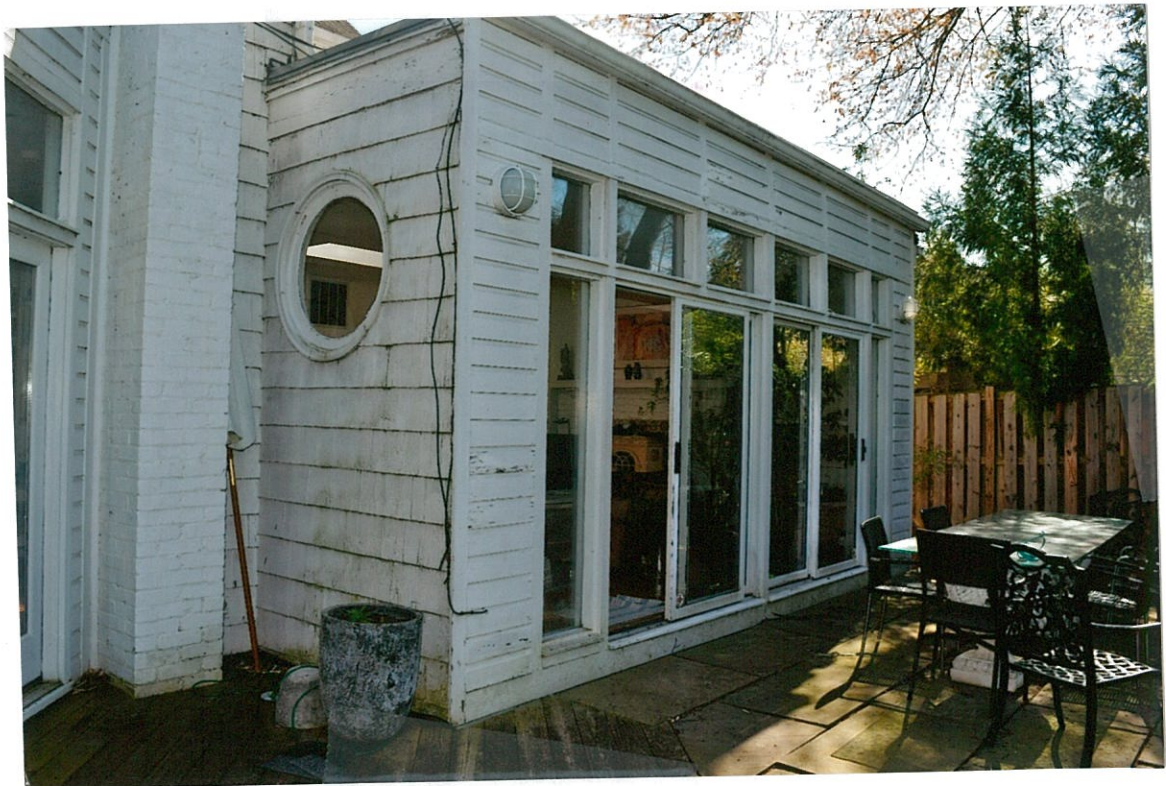
Detail Photo#22 4/25/18 Rear (north) elevation showing 1 st -floor ca. 1960 family room needing siding repairs, paint
