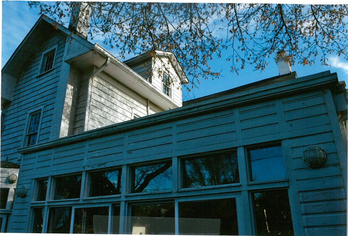
Detail Photo#25 4/25/18 Rear (north) elevation showing 1 st -floor ca. 1960 family room needing siding repairs, paint, plus part of 2 nd floor side (west) elevation
