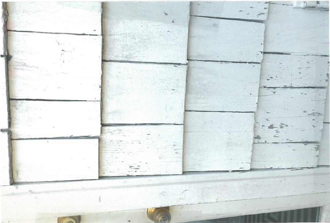
Detail Photo#46 8/22/18 side (east) elevation showing original cedar siding, removed years ago and repainted
