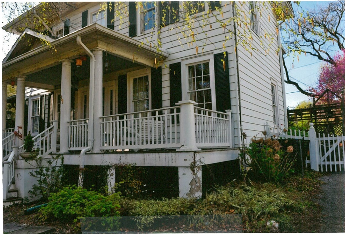
Detail Photo#13 4/25/18 Front (south) elevation side (east) elevation detail of front porch railing showing peeling paint, mildew
