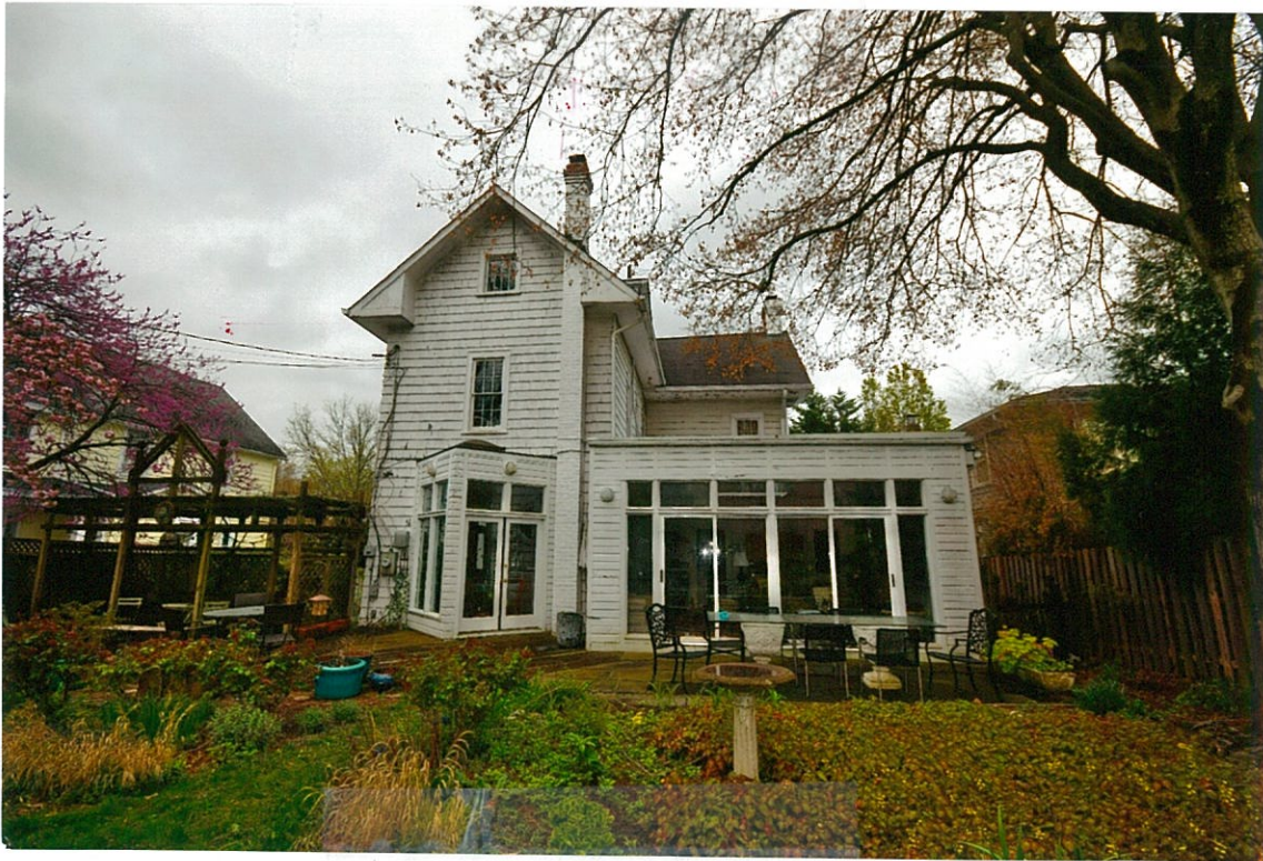
Detail Photo#20 4/25/18 Rear (north) elevation showing 3-story oldest part of house and ca. 1960 1-story family room
