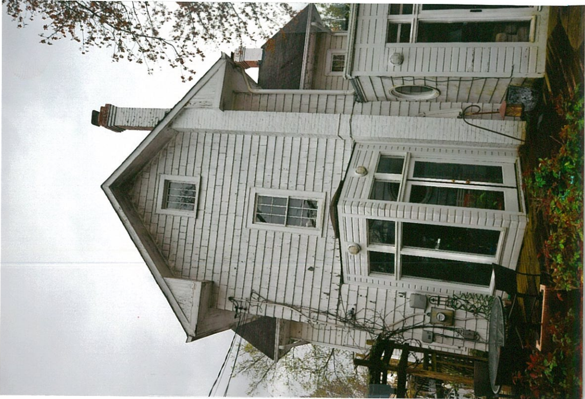
Detail Photo#23 4/25/18 Rear (north) elevation showing 3-story oldest part of house with original cedar shingles and adjoining 1-story ca. 1960 family room
