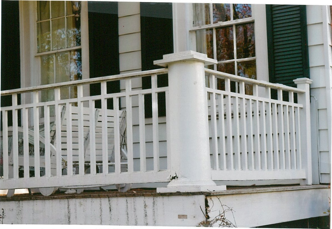
Detail Photo#12 4/25/18 Front (south) elevation Front (south) elevation and side (east) elevation detail of front porch railing
