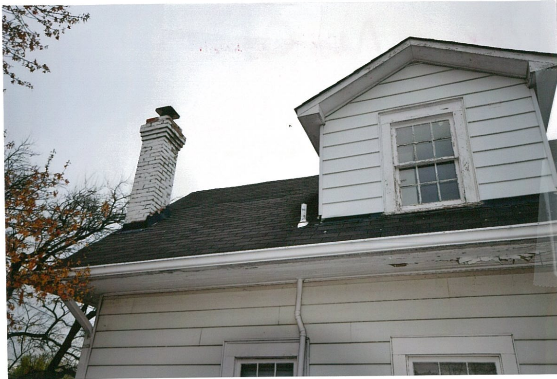
Detail Photo# 41 40 4/25/18 rear (north) elevation and side (west) elevation showing 2 nd floor exterior and family room roof, aluminum siding to be removed, eaves and woodwork needing painting
