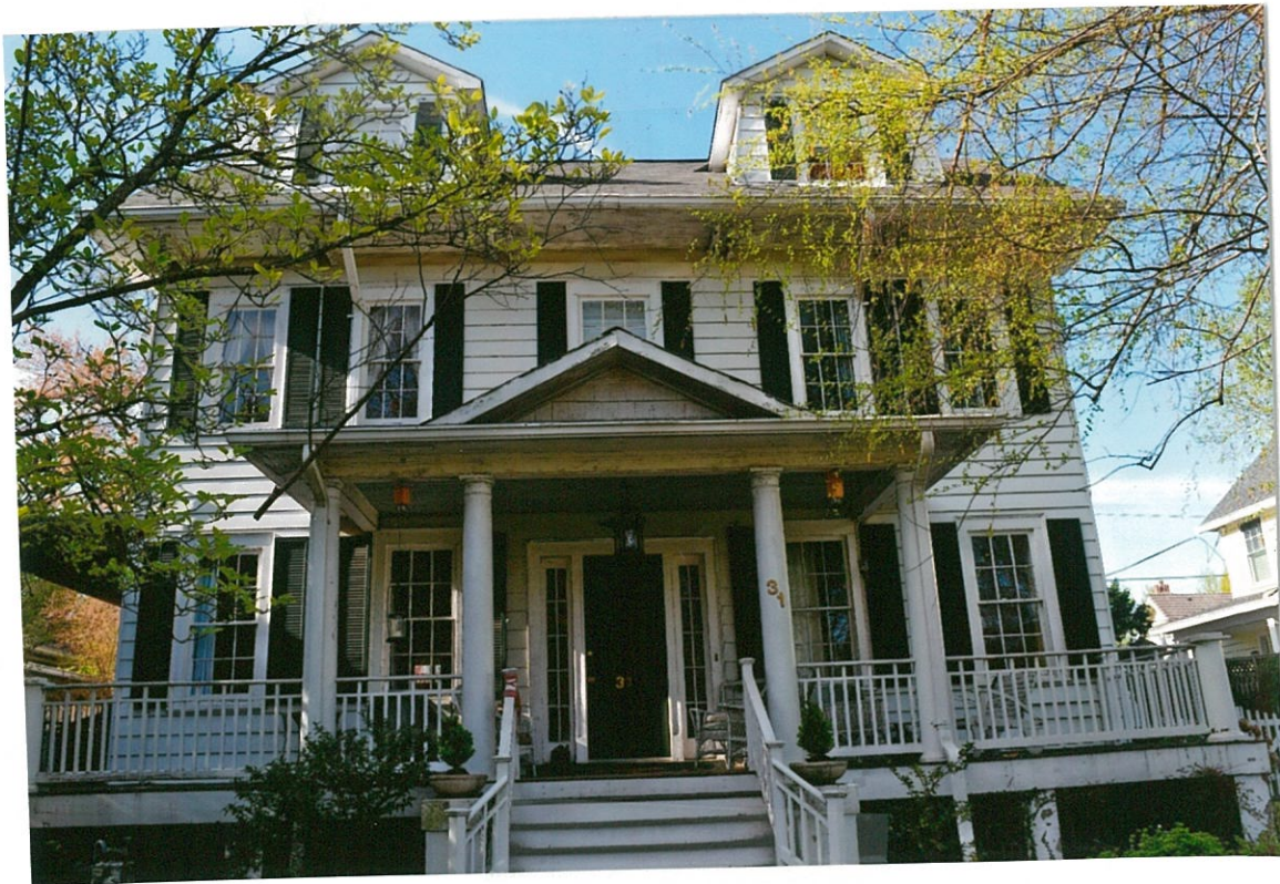
Detail Photo# 6 4/25/18 Front (south) elevation Shows mildew, peeling paint under eaves aluminum siding to be removed
