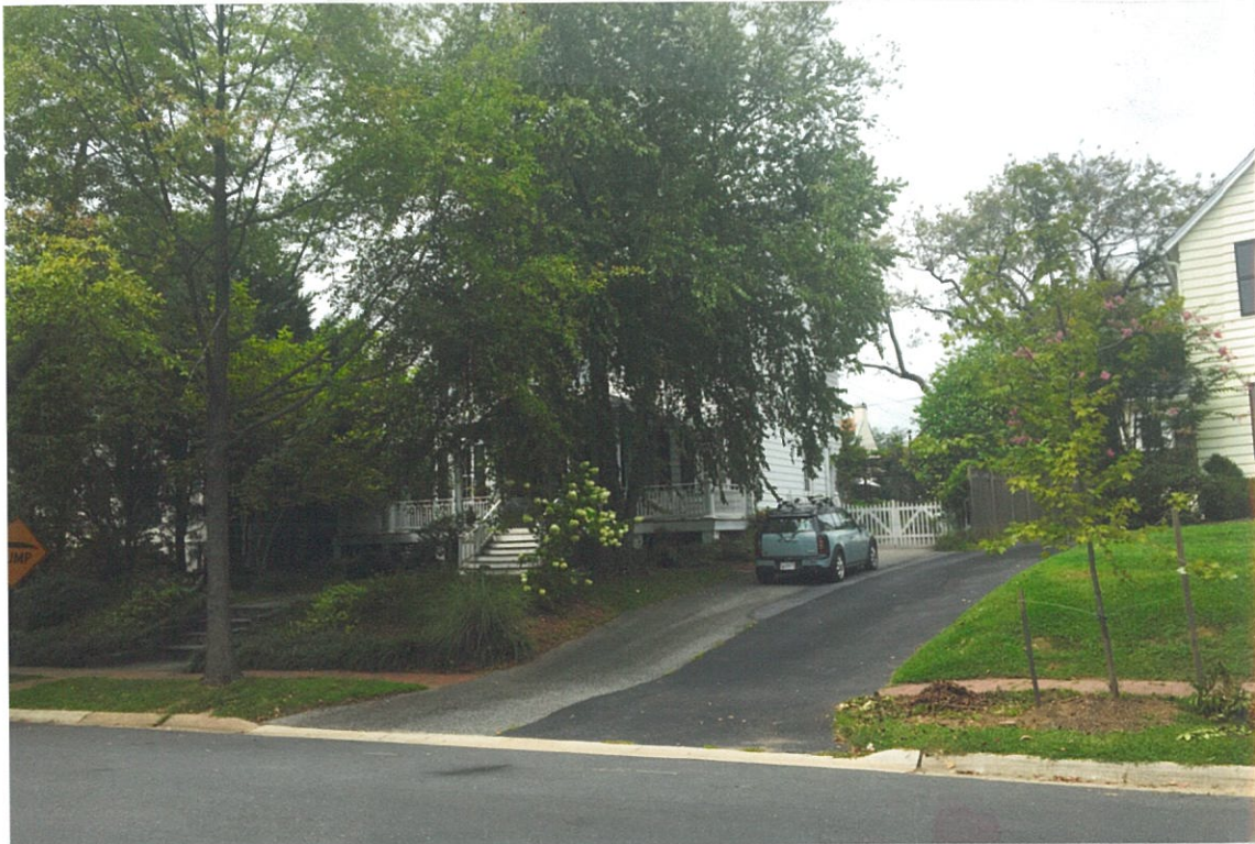
Detail Photo# 3 8/20/18 Front (south) elevation Shows view from adjacent neighbors at 33 Oxford Street
