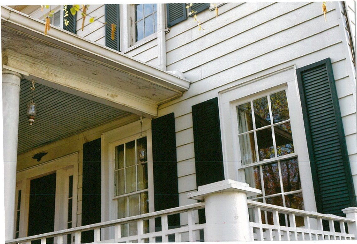
Detail Photo#15 4/25/18 Front (south) elevation Front (south) elevation, detail of front porch showing aluminum siding to be removed
