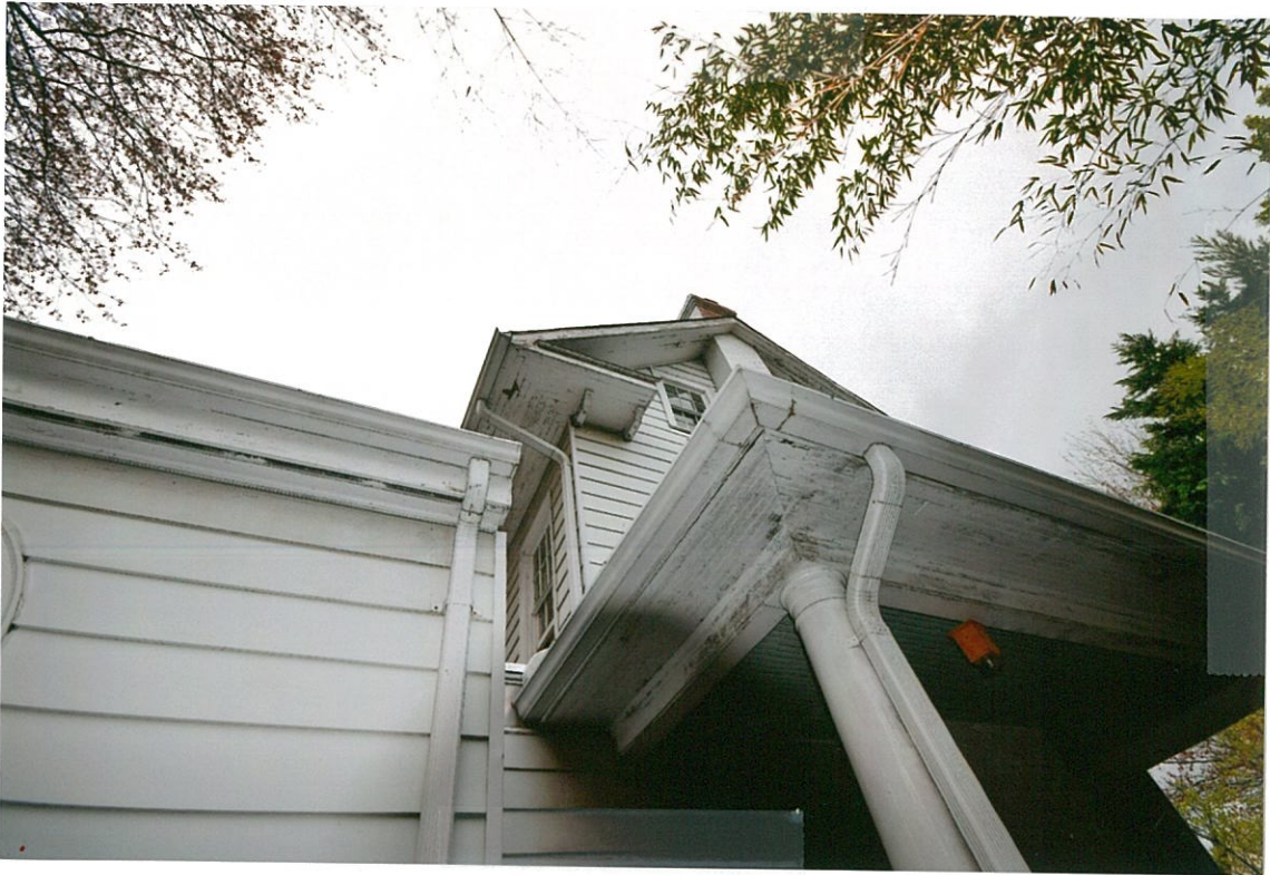
Detail Photo #37 4/25/18 Side (west) elevation showing exterior of family room and edge of wraparound front porch, showing aluminum siding to be removed, woodwork needing painting
