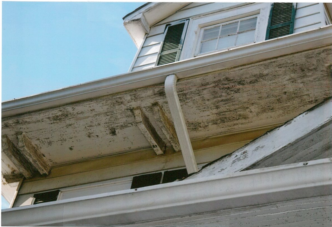
Detail Photo# 10 4/25/18 Front (south) elevation Front (south) elevation detail of eaves with peeling paint, mildew
