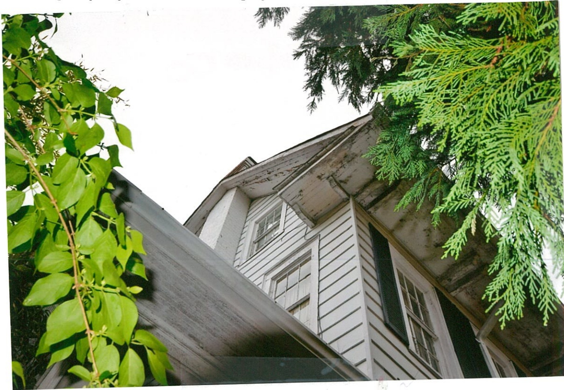
Detail Photo#17 4/25/18 Front (south) elevation Front (south) elevation, detail of 2 nd and 3 rd floor eaves shot from front yard
