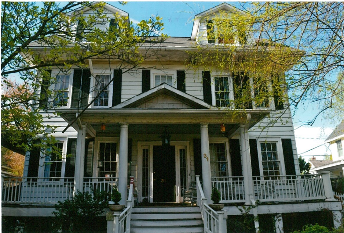
Detail Photo# 2 4/25/18 Front (south) elevation Shows mildew, peeling paint, aluminum siding to be removed
