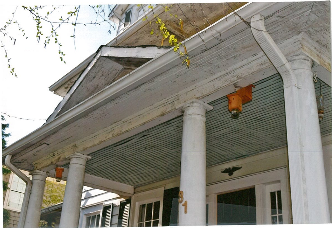
Detail Photo# 9 4/25/18 Front (south) elevation Front (south) elevation detail of covered front porch Shows peeling paint, mildew
