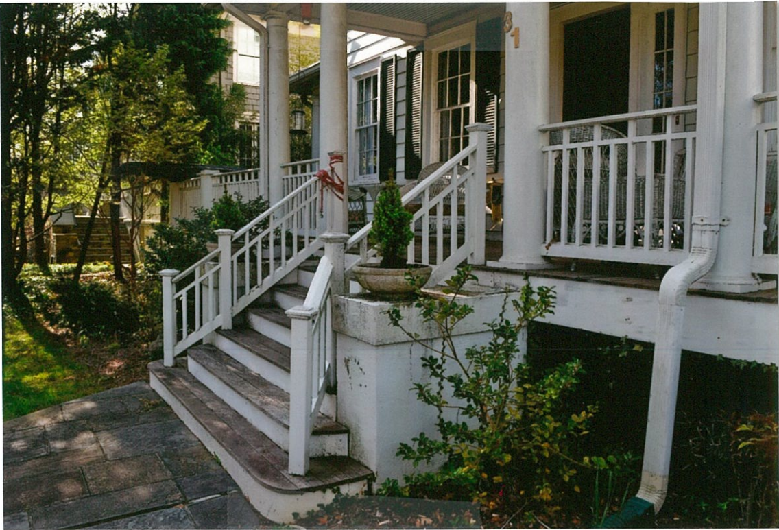
Detail Photo#11 4/25/18 Front (south) elevation Front (south) elevation detail of front steps and railing Shows peeling paint, mildew
