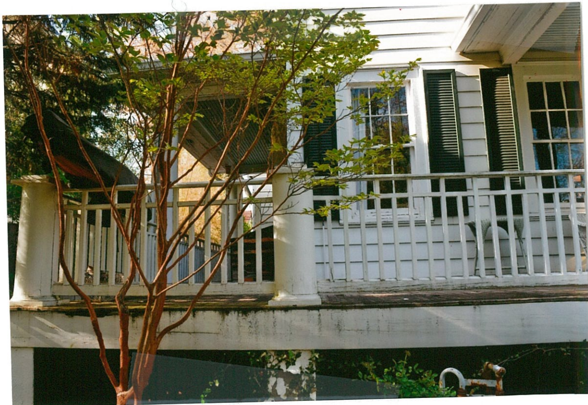
Detail Photo#16 4/25/18 Front (south) elevation Front (south) elevation, detail of front porch showing aluminum siding to be removed
