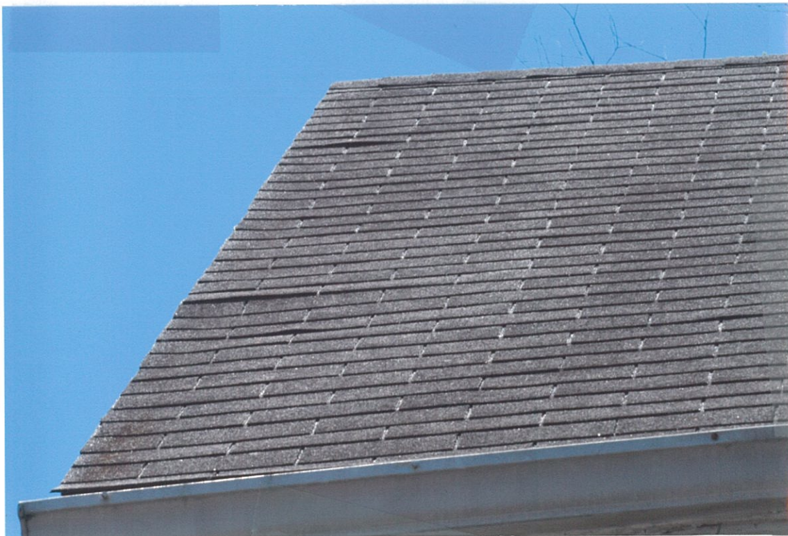
Detail Photo#43 rear (north) elevation roof showing missing and irregular shingles
