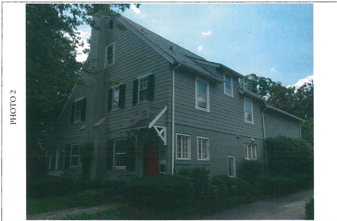
Detail: FRONT/RIGHT SIDE OF HOUSE - PORCH WILL NOT BE VISIBLE. IT WILL BE OBSCURED BY THE PREVIOUS REAR ADDITION
