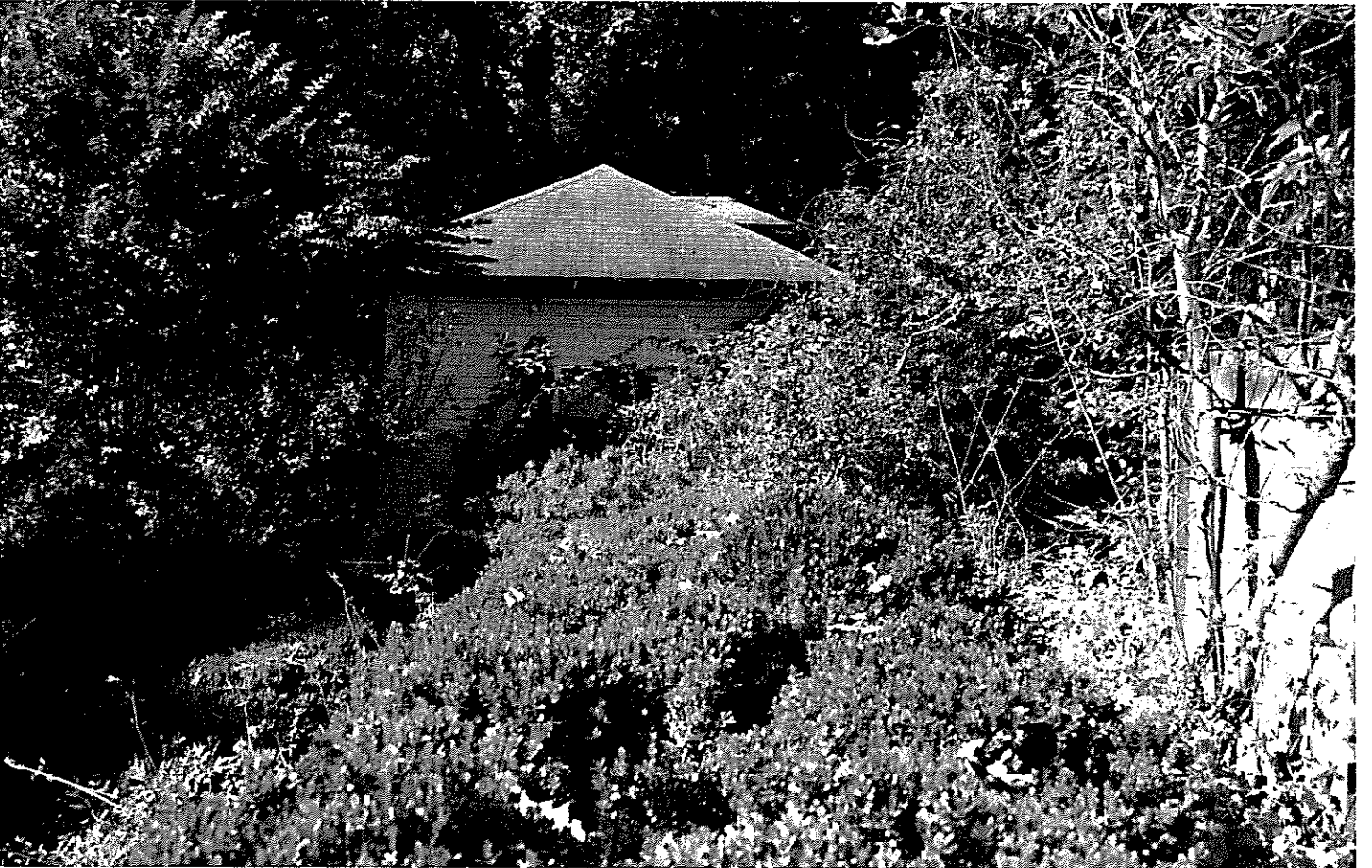
Existing garage East elevation
