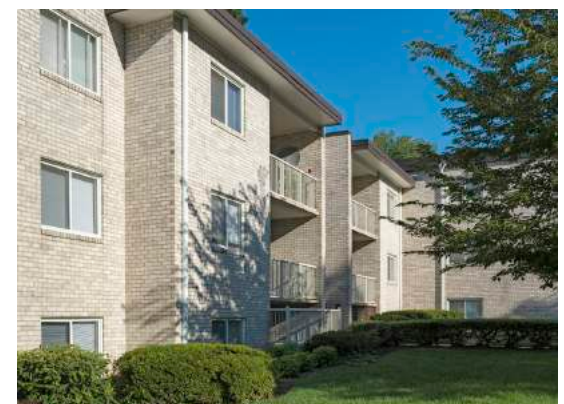
Existing multifamily residential. From top: The Monterey Apartments; Midtown Condominiums, Oxford Square Apartments.
