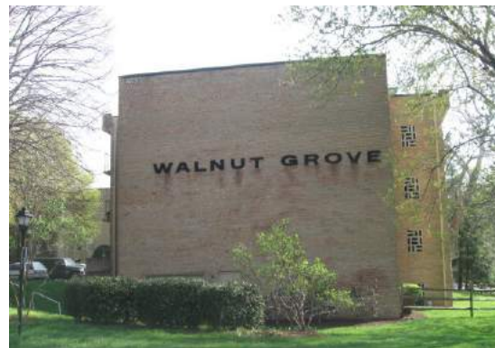
Existing uses: Loehmann's Plaza (top), Walnut Grove Condominiums (bottom).
