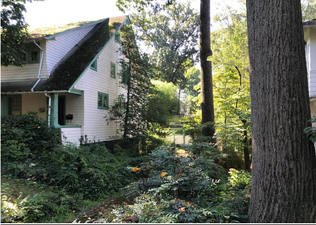
Figure 3: The right elevation of the house as viewed from the adjacent sidewalk.
