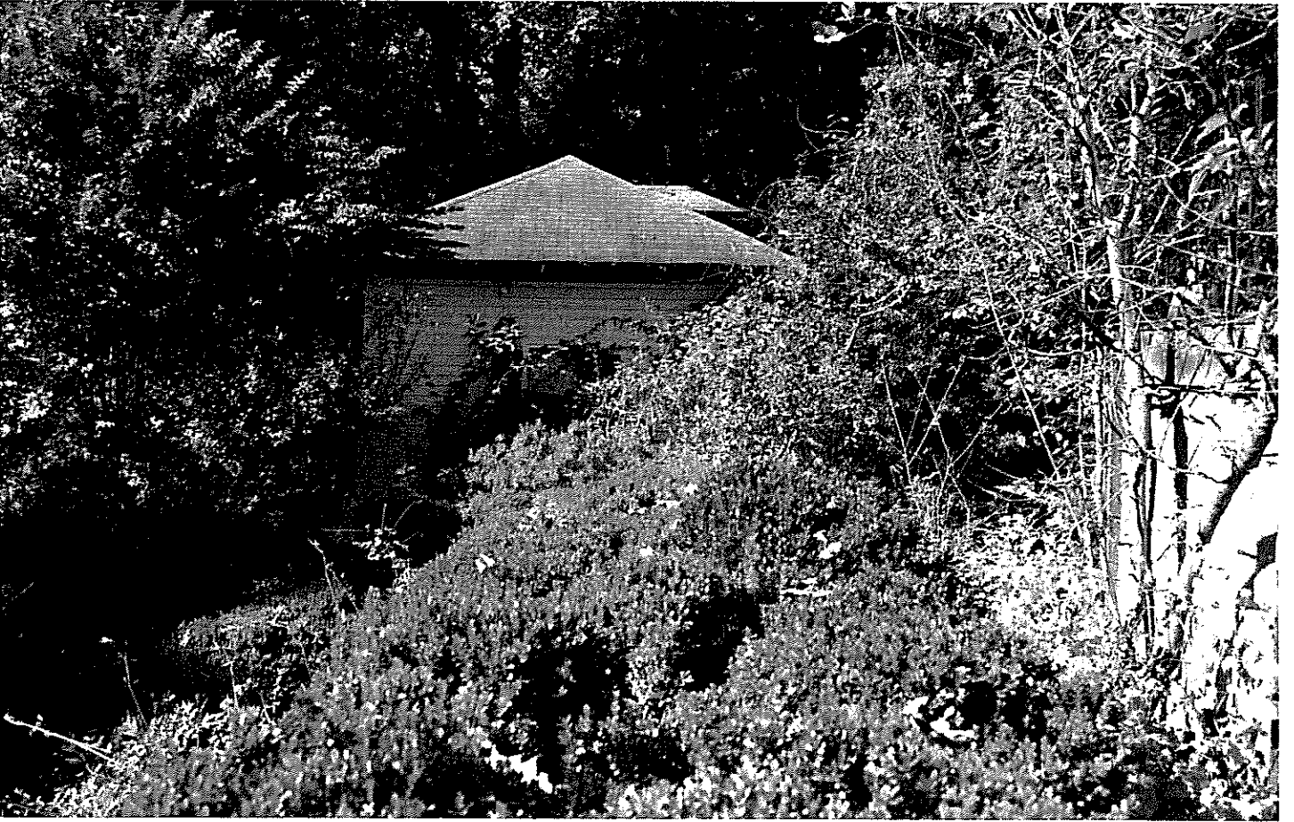
Existing garage East elevation
