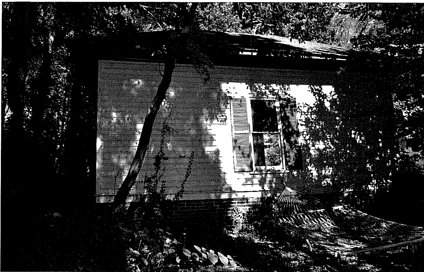
Existing garage South elevation
