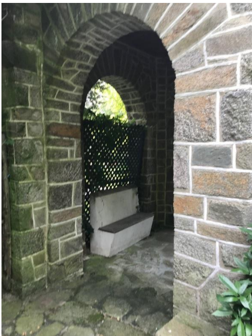
Figure 5: View of the gazebo looking through the north and east openings.
