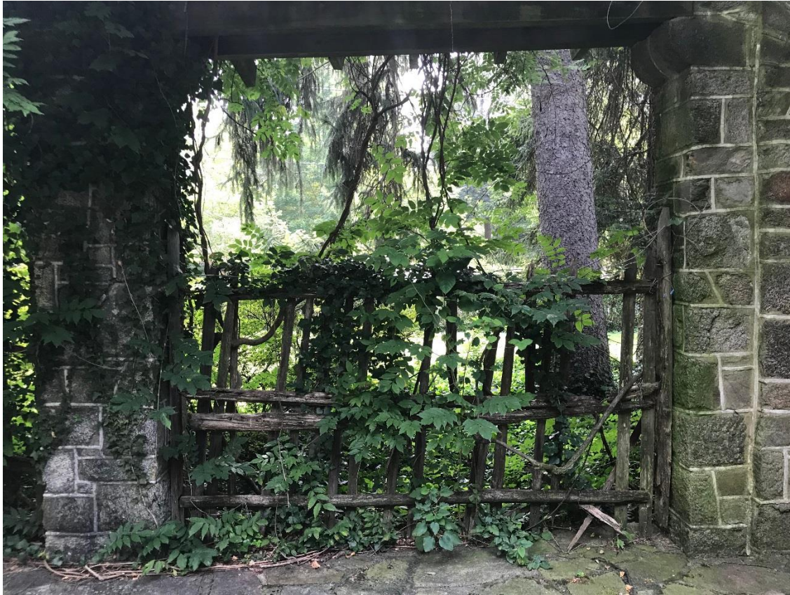
Figure 4: Columns supporting the pergola with fencing and vines between the columns.
