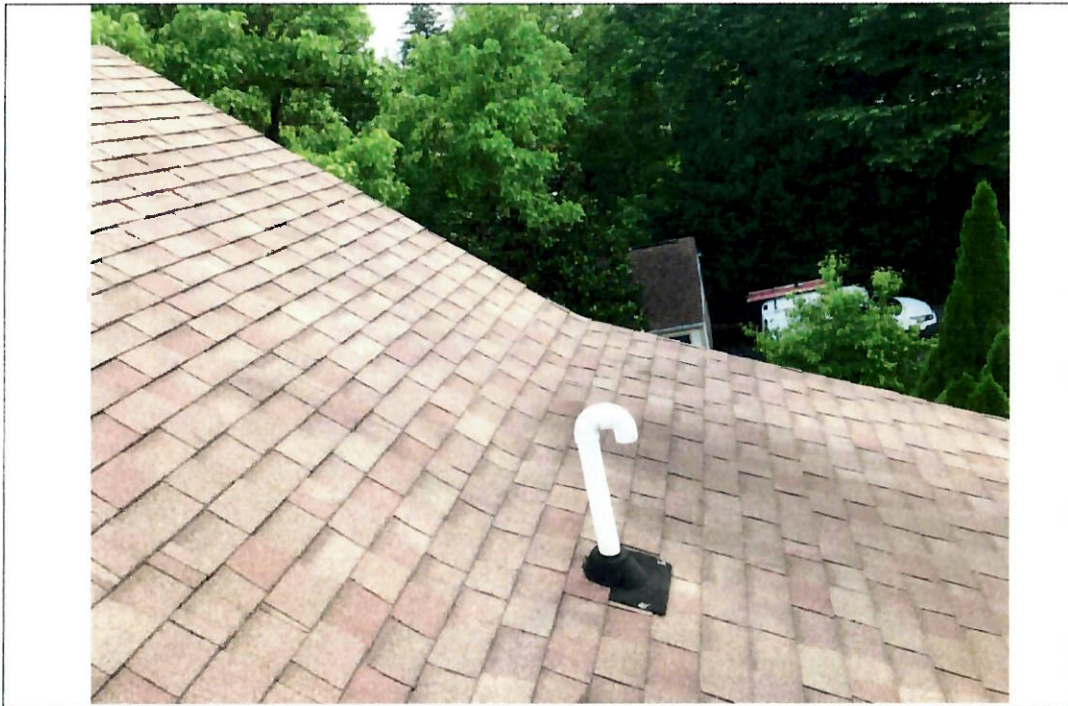
Detail: on mounting plane MP1, facing rear of home MP2B
