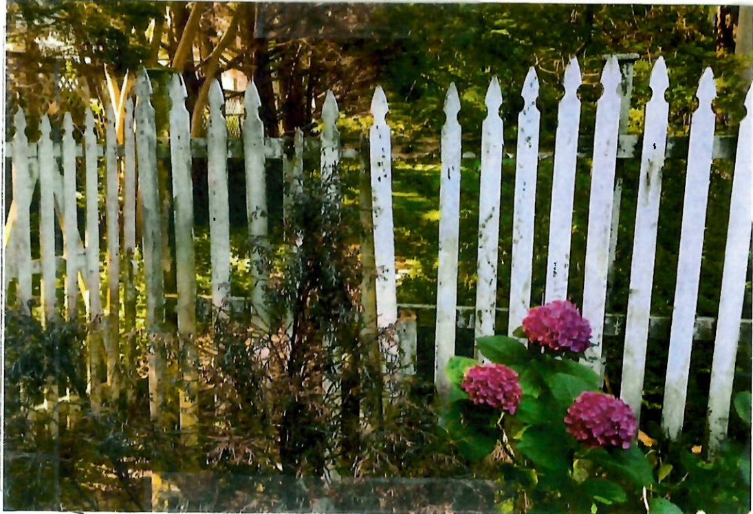
Detail: DETAIL OF FENCE - FROM GATE WEST TO PORCH
