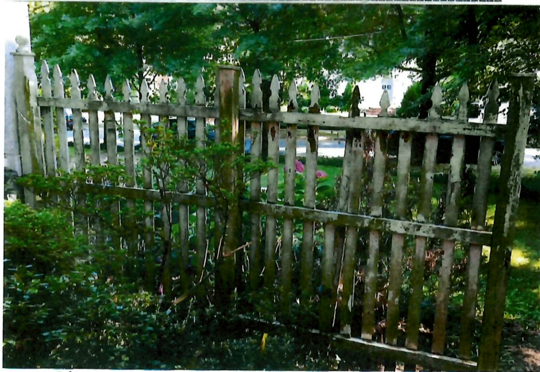
Detail: BACK OF FENCE FROM PORCH TO GATE - SOUTH LOOKING NORTH
