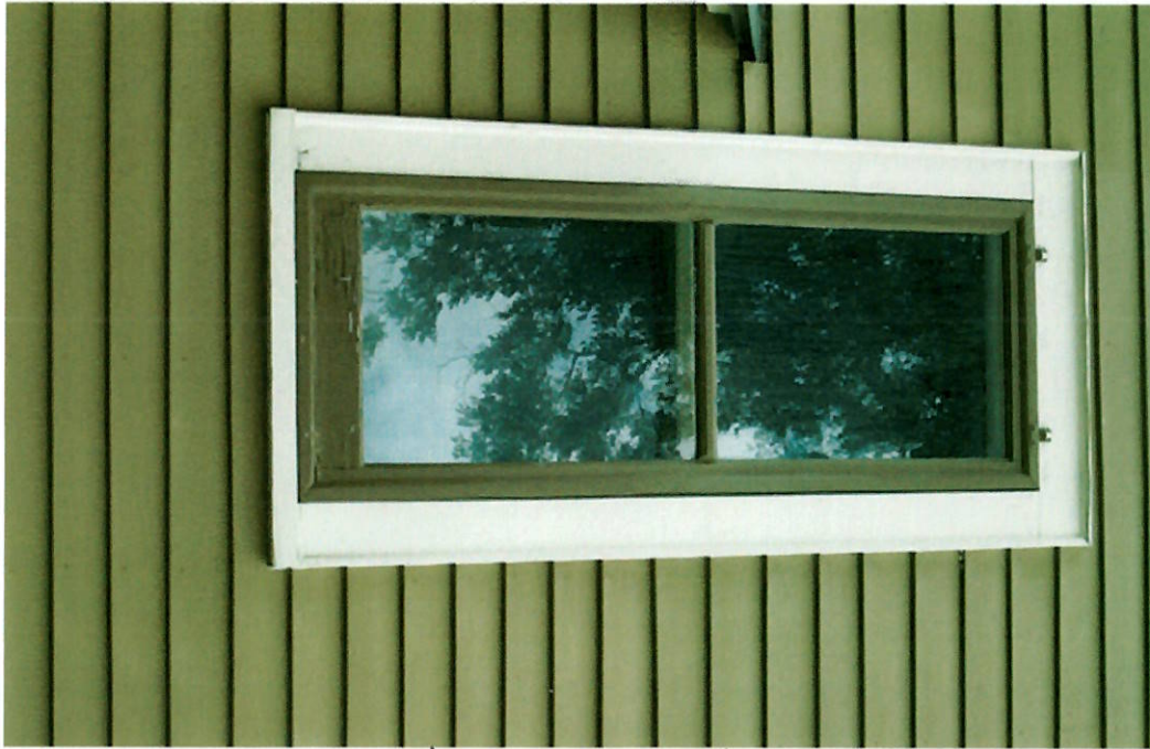
wood storm window - typical condition
