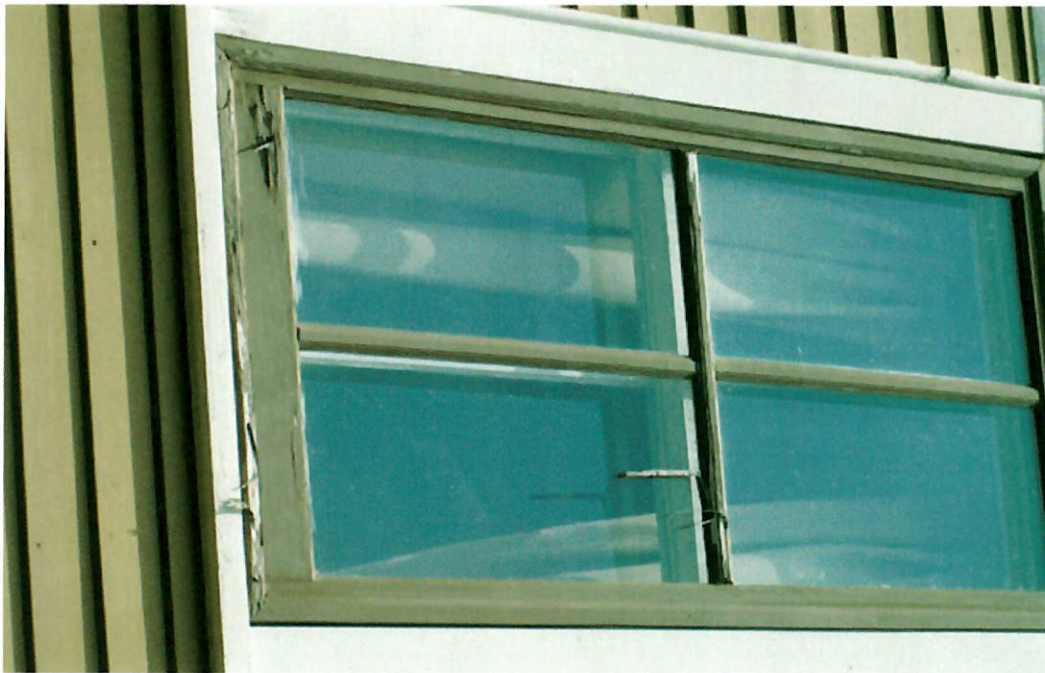
wood storm window - typical condition
