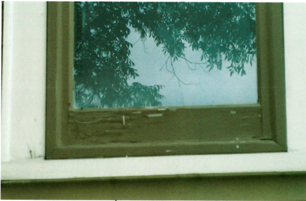
wood storm window - typical condition
