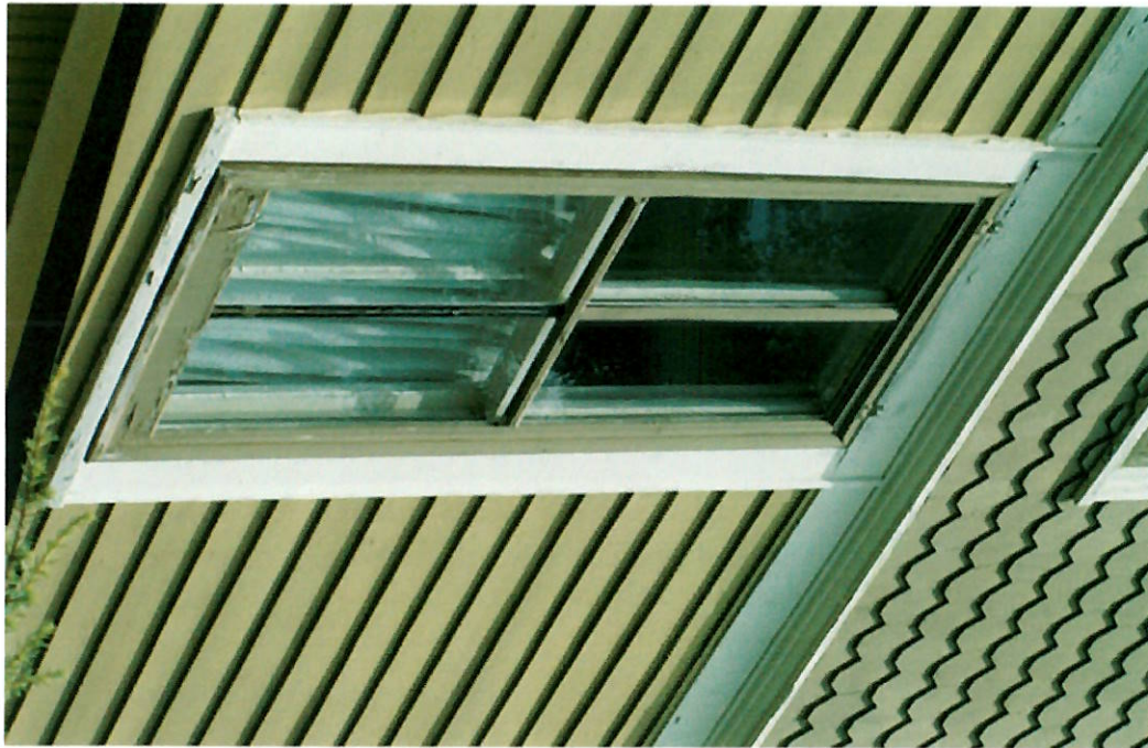
wood storm window - typical condition
