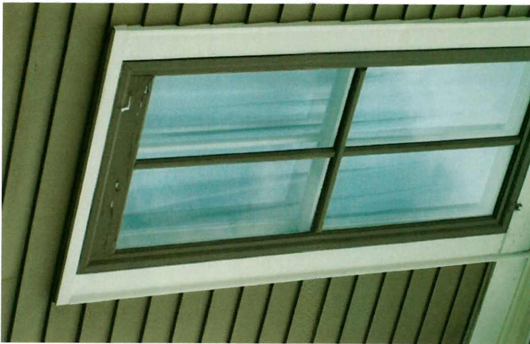
wood storm window - typical condition
