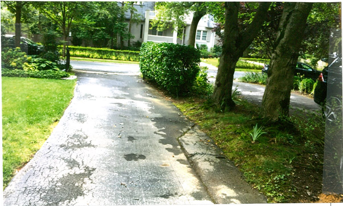
Detail: Two maple trees on property line 3' from DRIVEWAY
