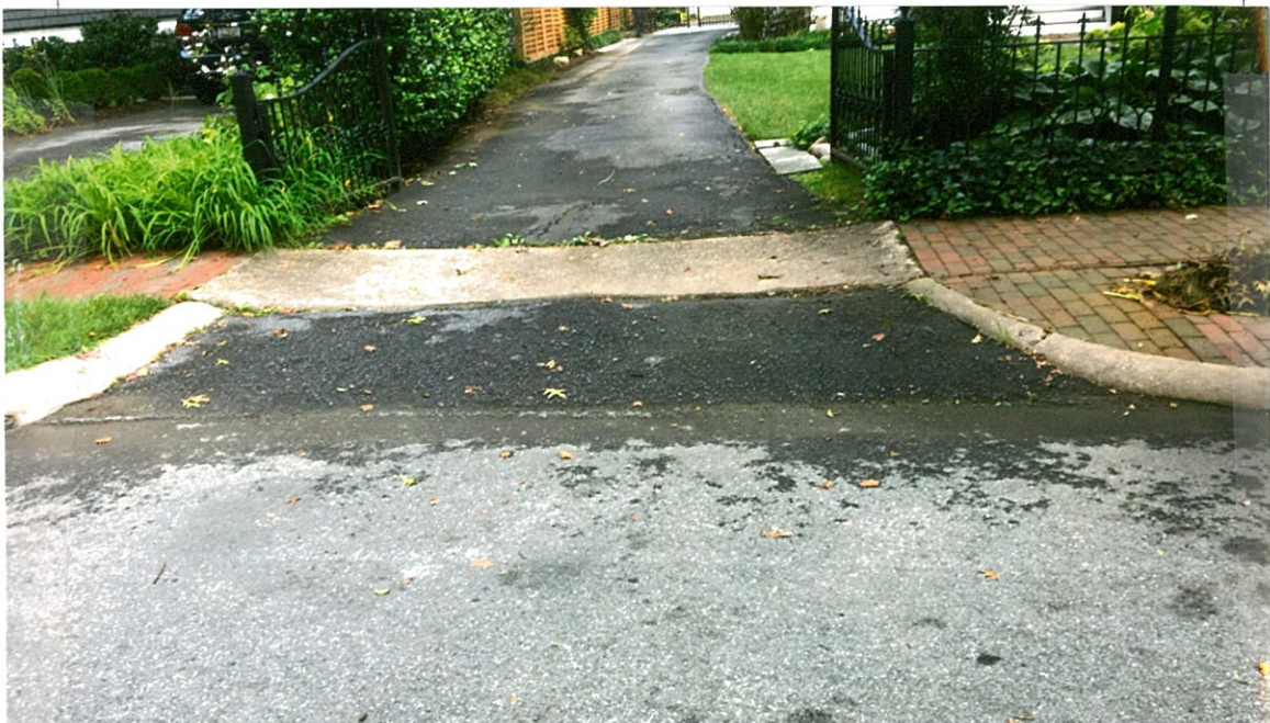
Detail: Apron from Newlands St to driveway
