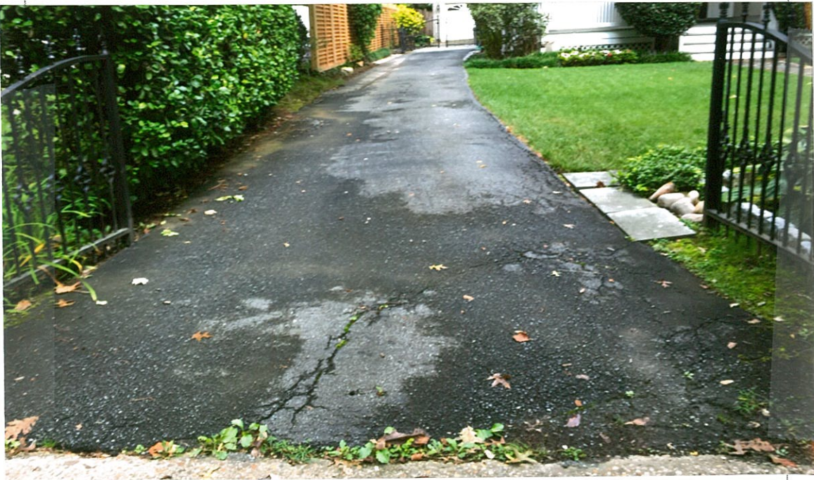
Detail: FROM SOUTH LOOKING NORTH
