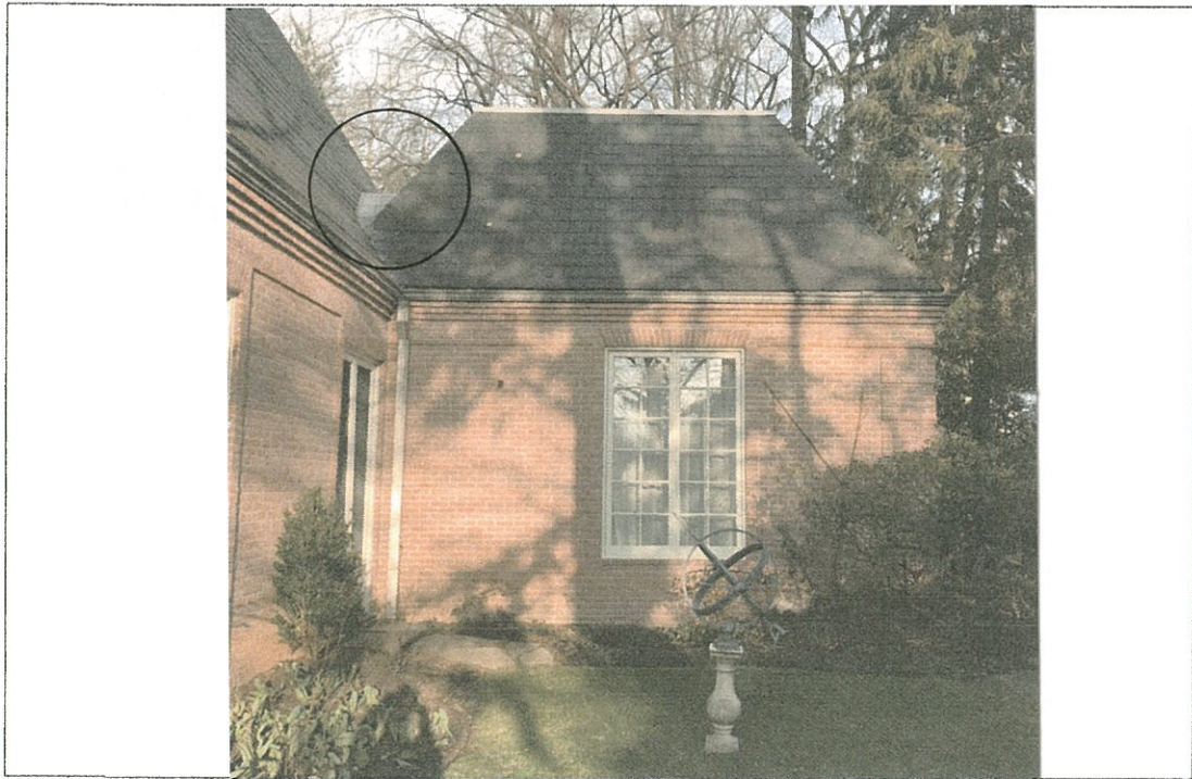
Detail: Location of existing cricket which will be made steeper.
