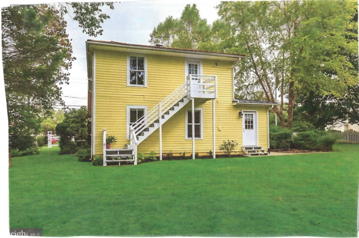
Detail: Rear View of House
