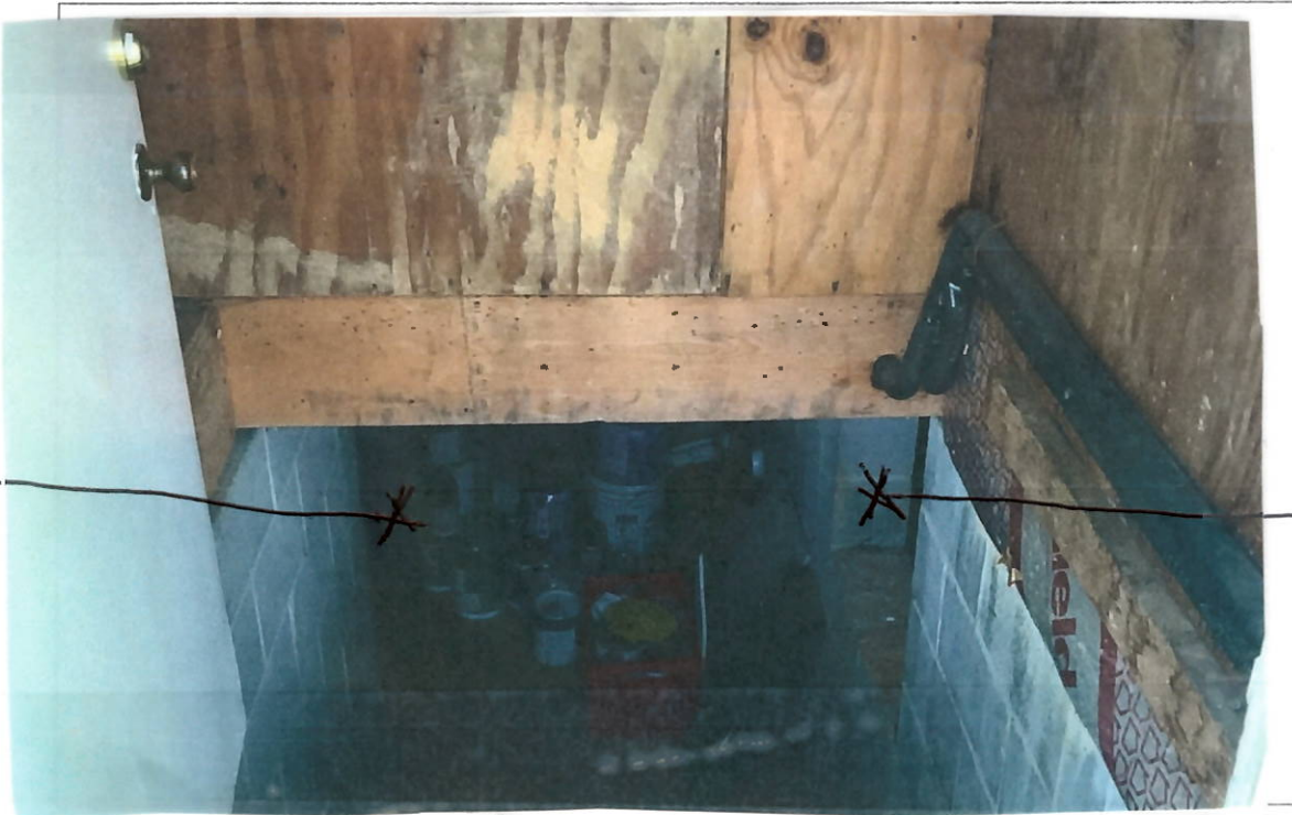
Detail: Entry to basement - only access is this door
