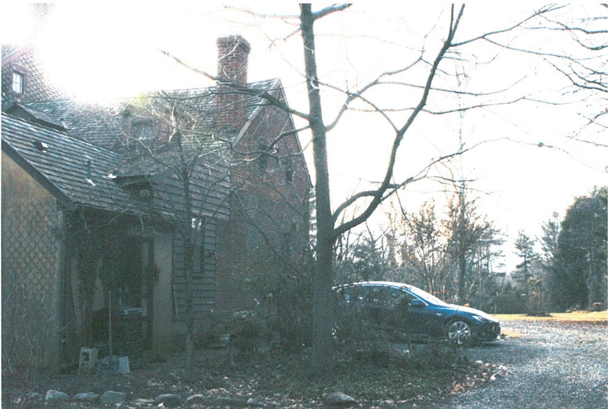
6 North facade, non historic portion. Shows location of new porch roof, non-historic siding to be replaced and stucco to be covered with siding.
