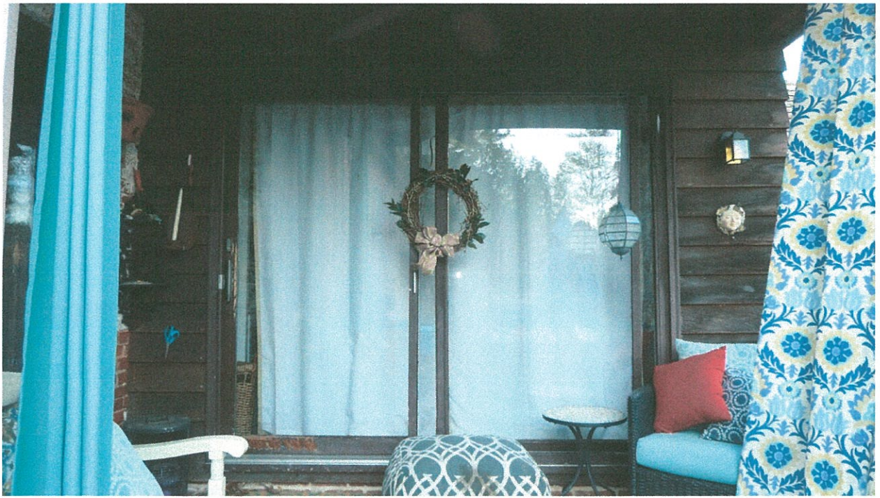
9 Slider (Door E) to be replaced.
