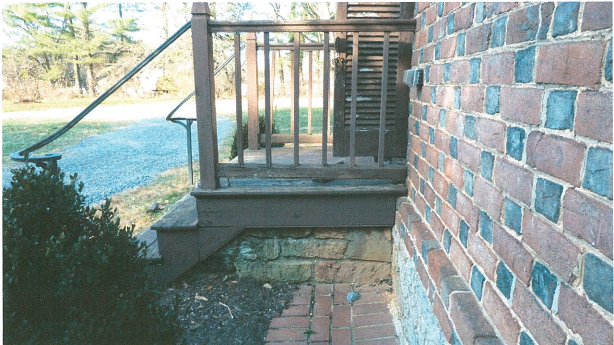
14 Main porch, side view
