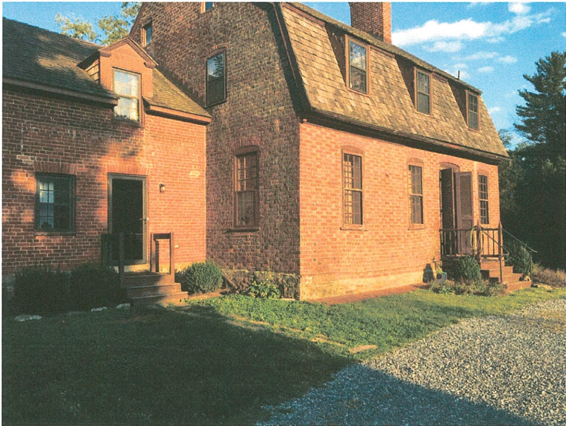
3 Main facade showing two non-historic porches to be replaced.
