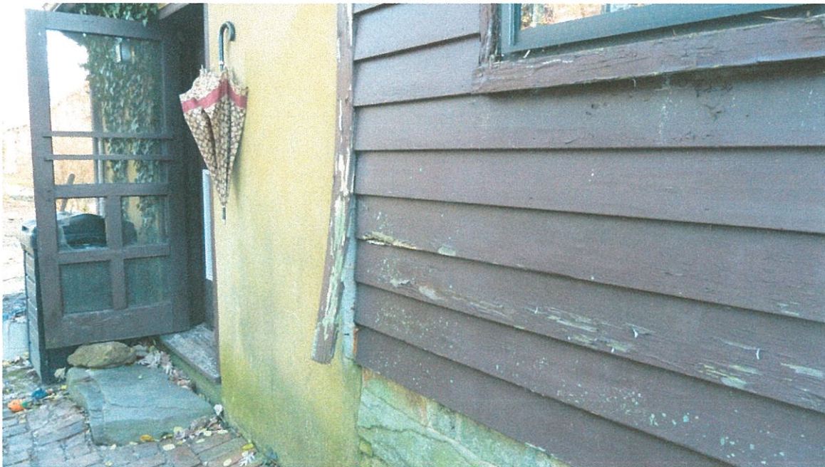
12 Non historic siding to replace with HardiePlank. Stucco to be sided to match.
