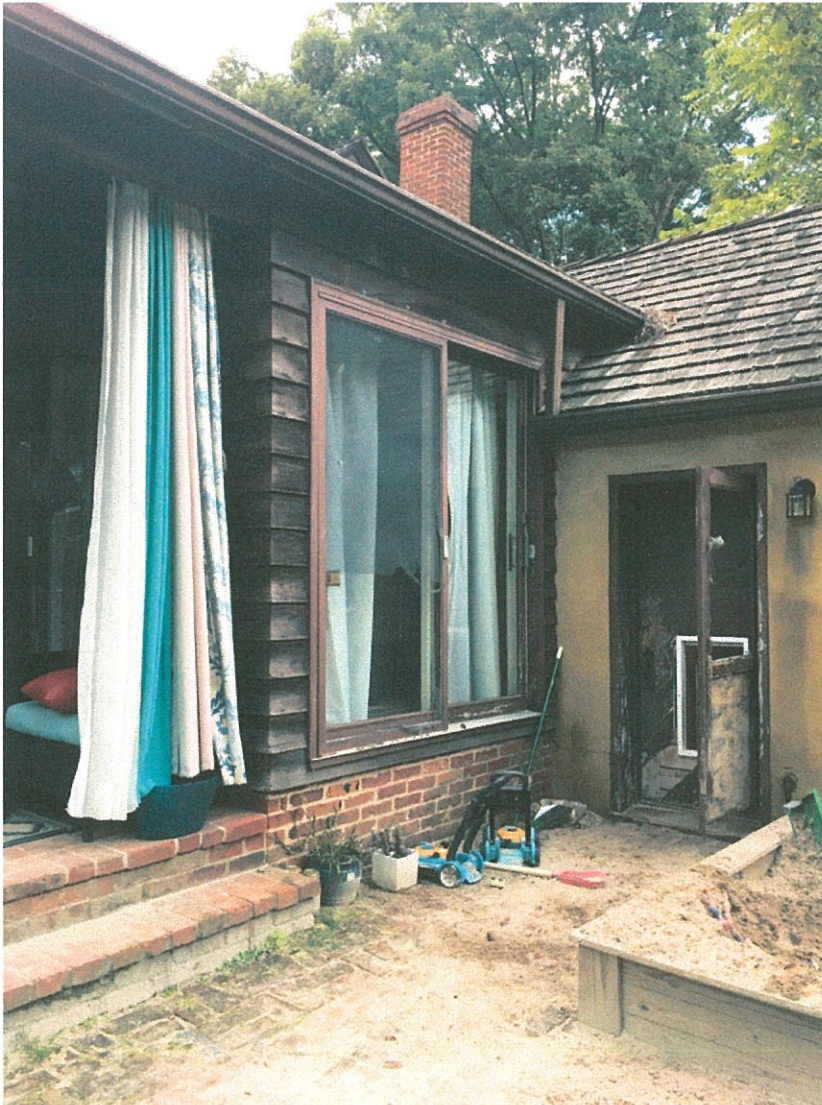
10 Slider (Door F) to be replaced with picture window. Siding to be replaced with HardiePlank. Stucco to be covered with Hardieplank.
