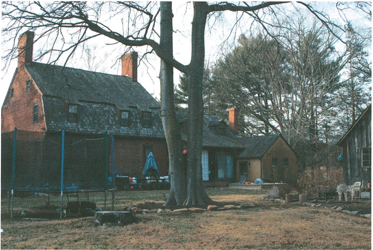
7 Rear (East) facade showing stucco addition and slider to be replaced with picture window.
