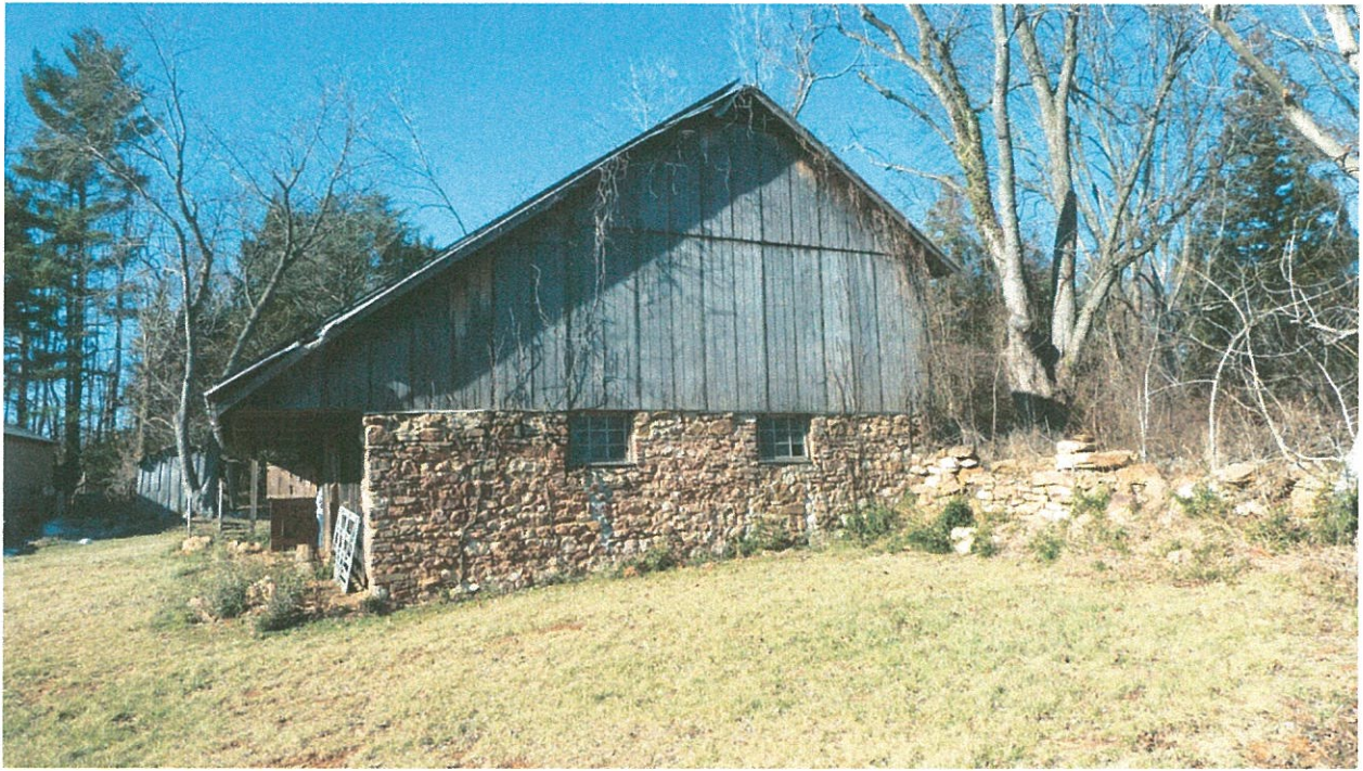
19 East facade with patched crack under window
