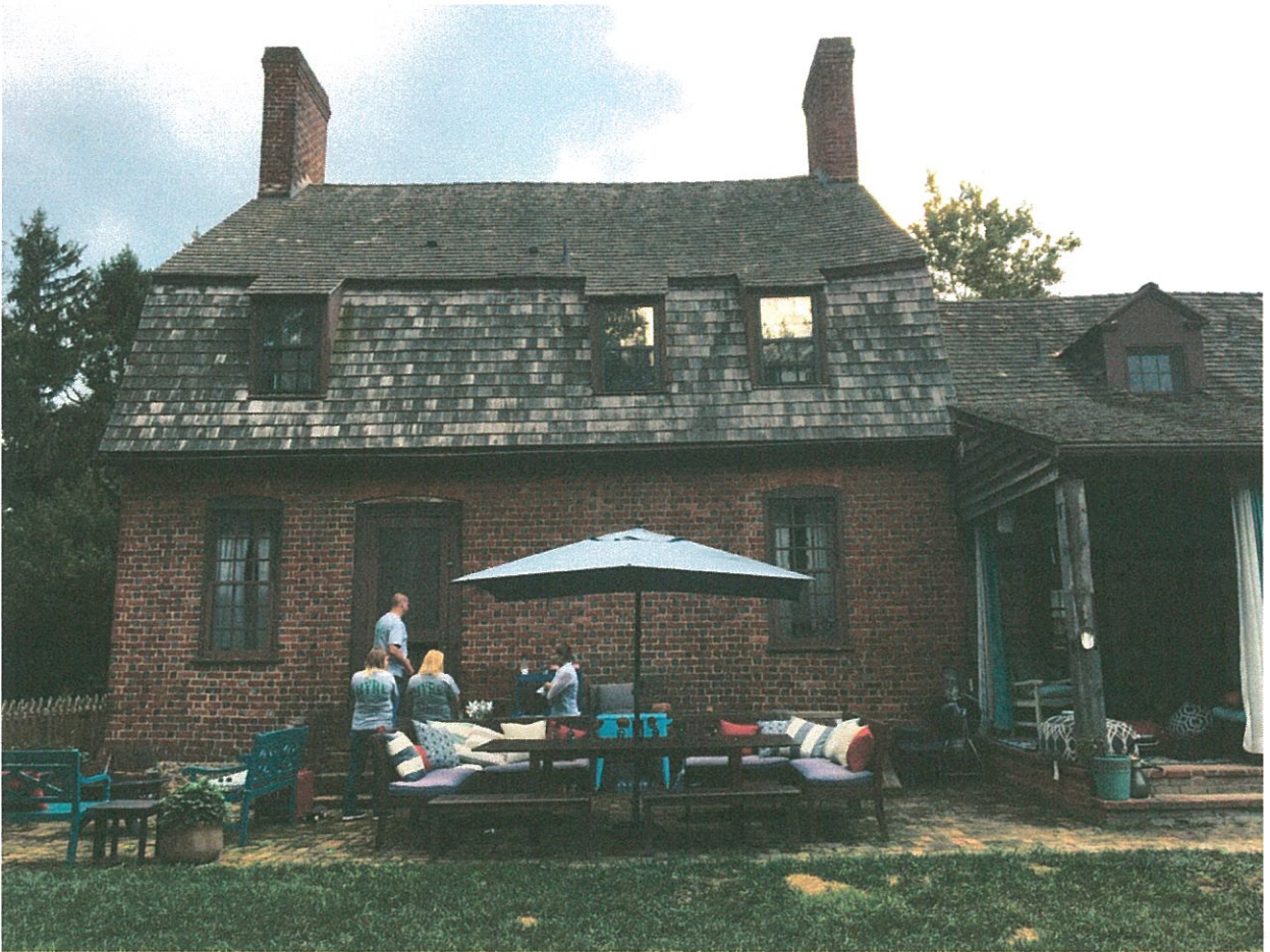
8 Rear facade, historic portion. Door C to be repaired and siding to be replaced. Windows and dormers to be repainted.
