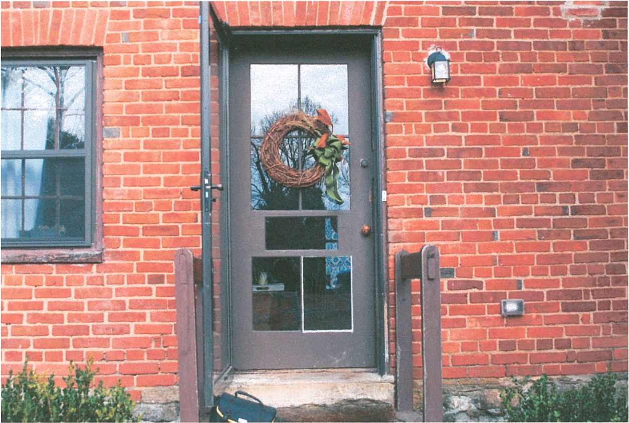
16 Secondary front porch, existing door to be replaced.
