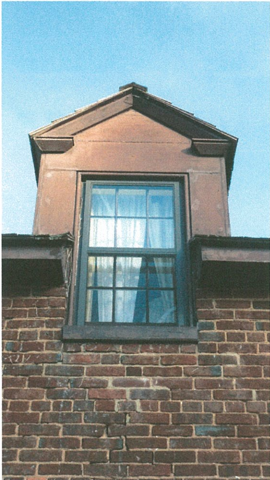
4 Brick repointing and dormer repainting work needed.
