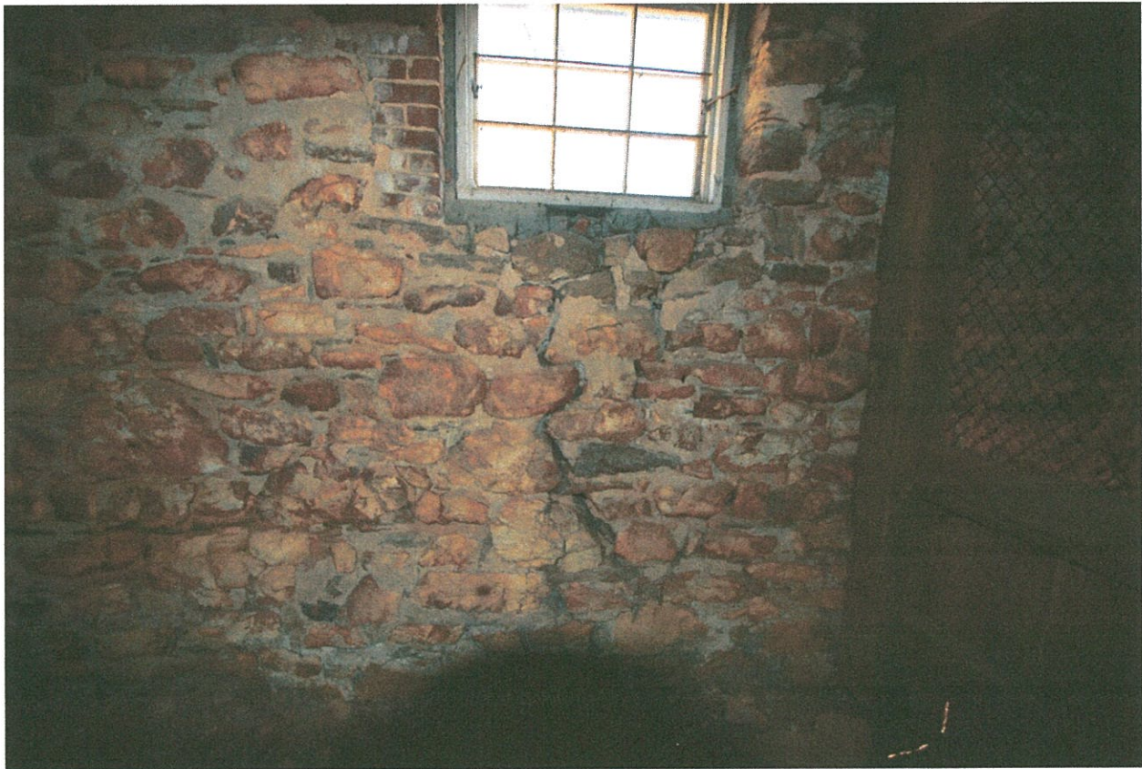
22 Interior of foundation wall crack
