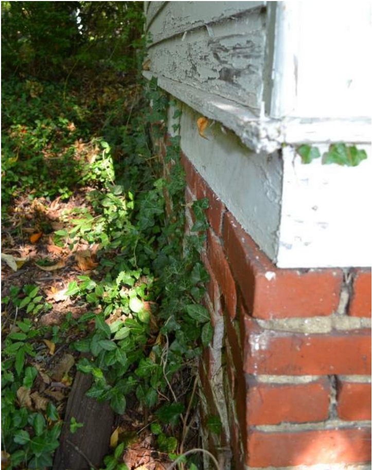
Existing garage foundation
