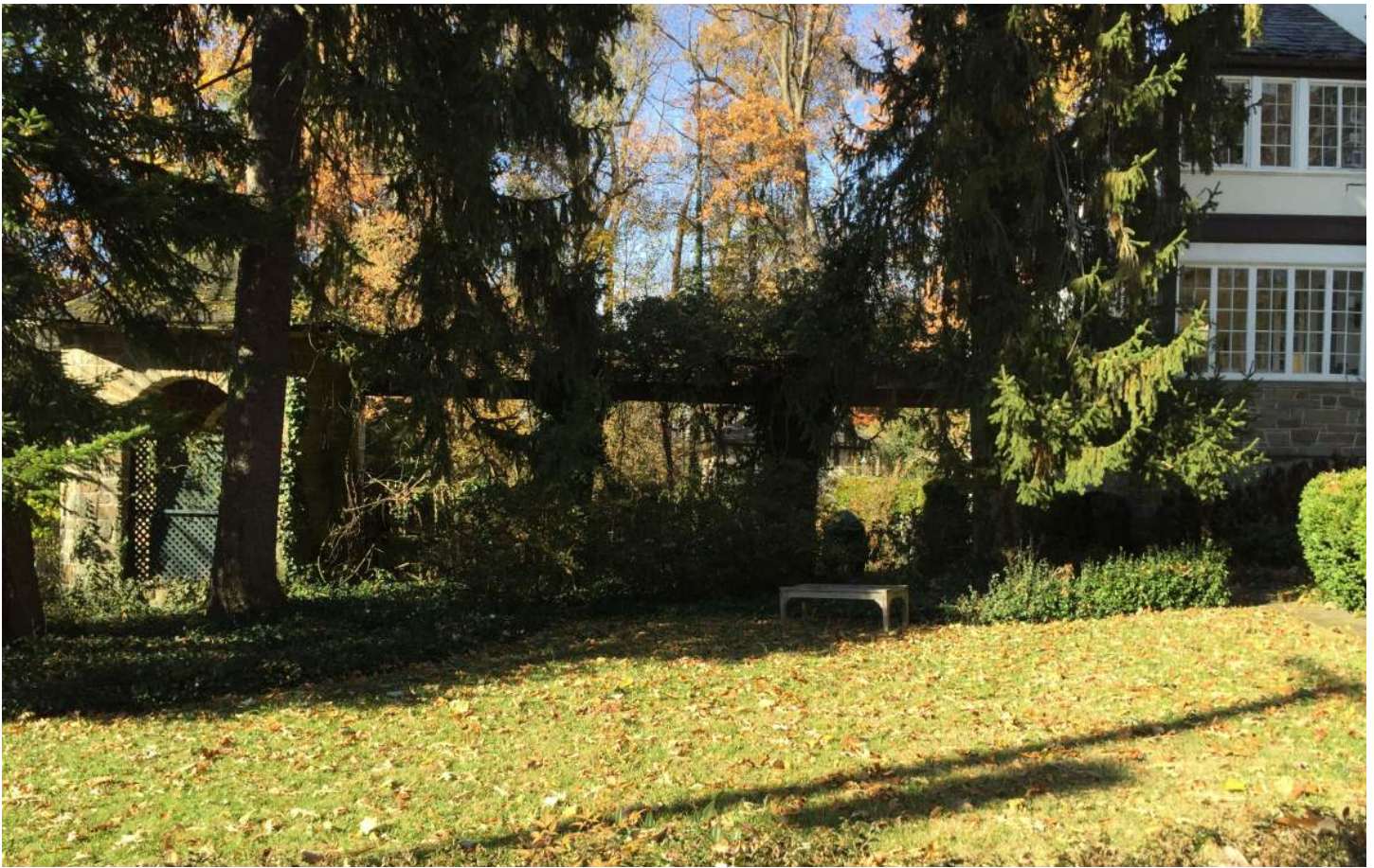
Existing pavilion & trellis from Cedar Parkway
