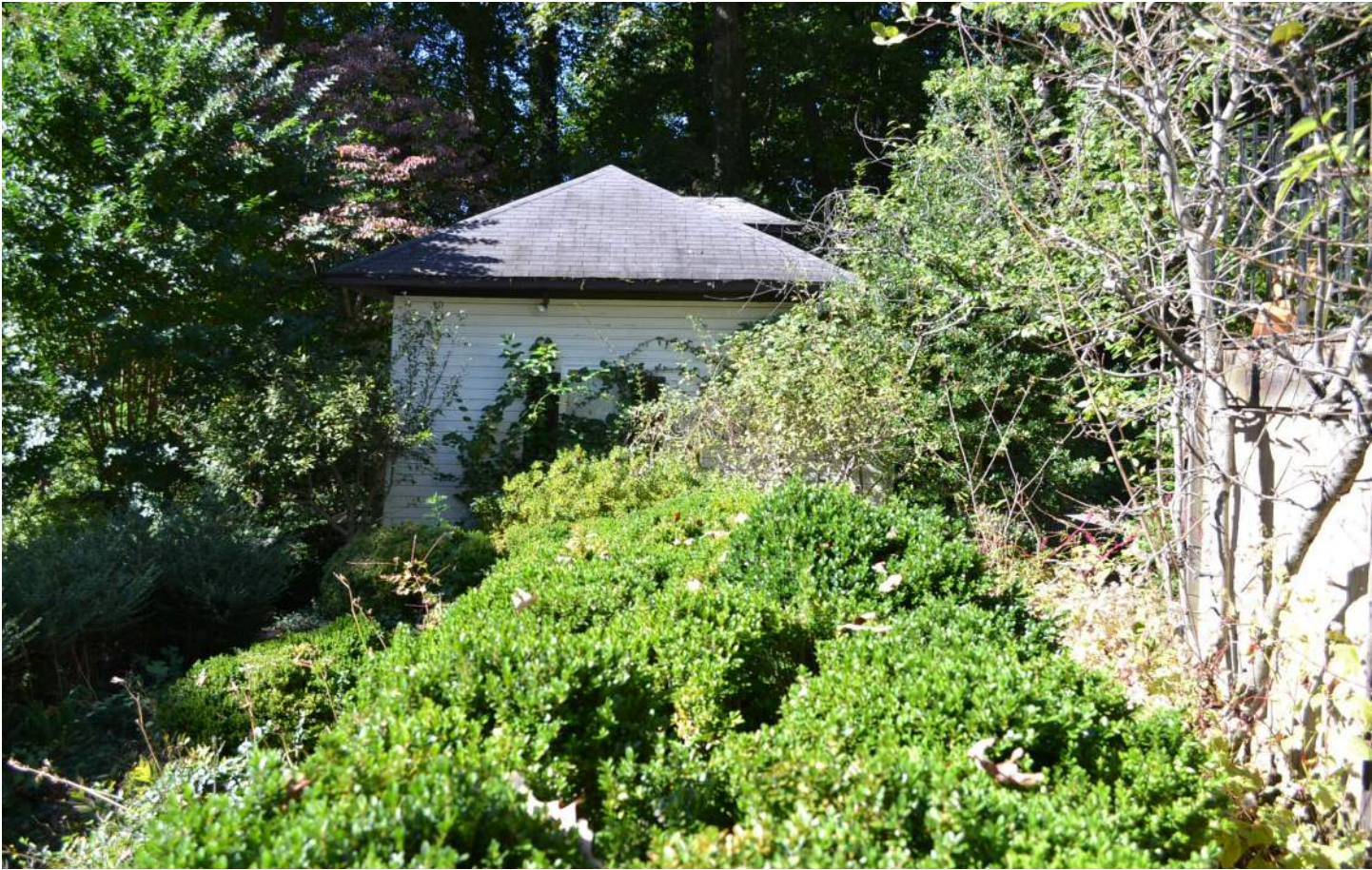
Existing garage East elevation
