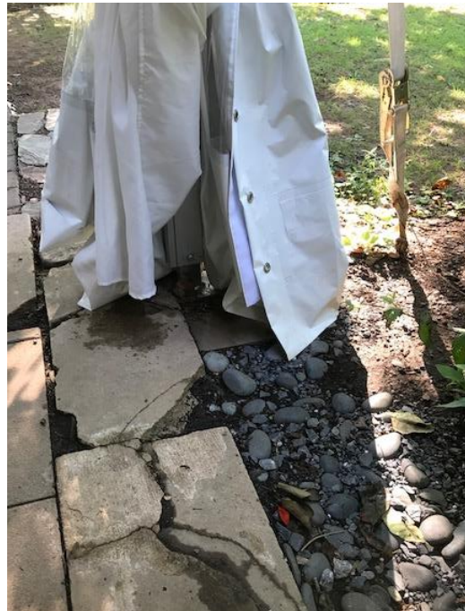
Southeast corner tent support and broken patio edging
