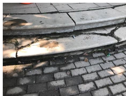
Crumbling stairs in the center of the patio leading to the lawn
