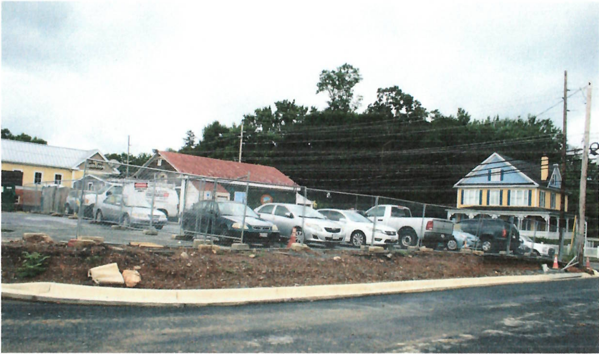
Existing site condition looking south from new Clarksburg Square Road
