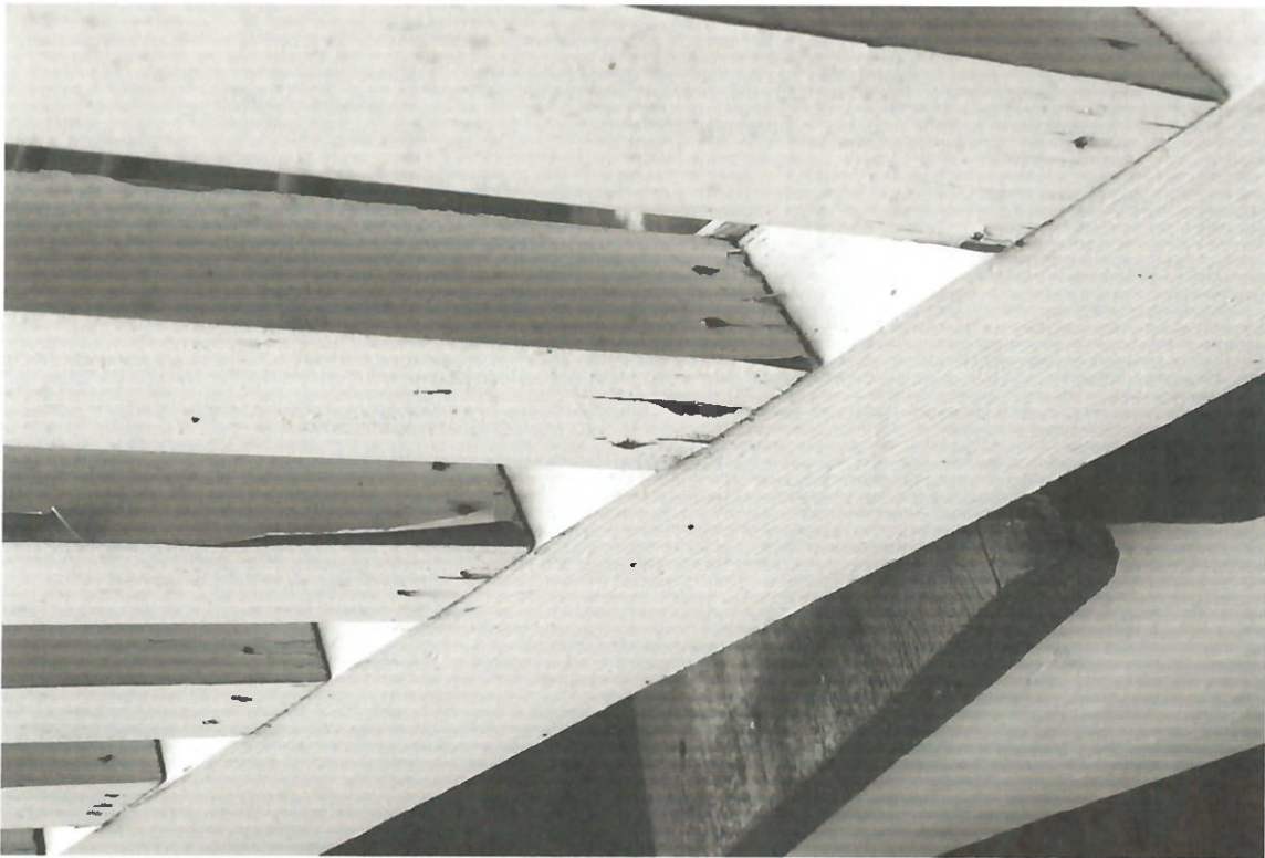
WOOD STAIRS AND RAILINGS TO BE REPLACED
