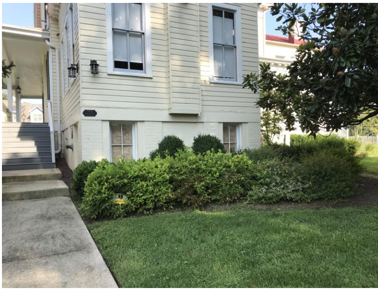
Figure 2: Crawlspace in the historic massing of the house showing the non-historic windows with the plywood behind.
