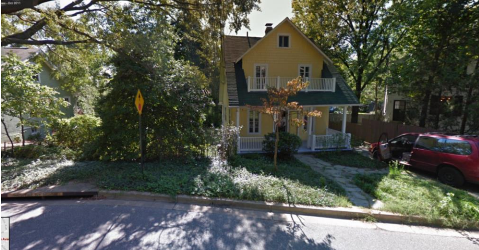
Figure 2: House and side yard showing the drop off and significant vegetation.
