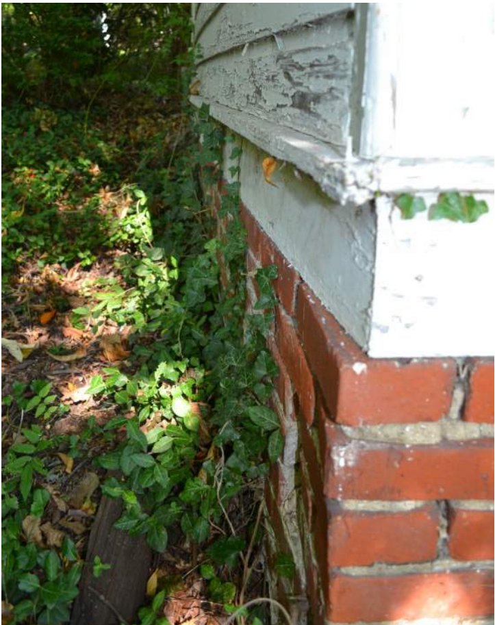
Existing garage foundation
