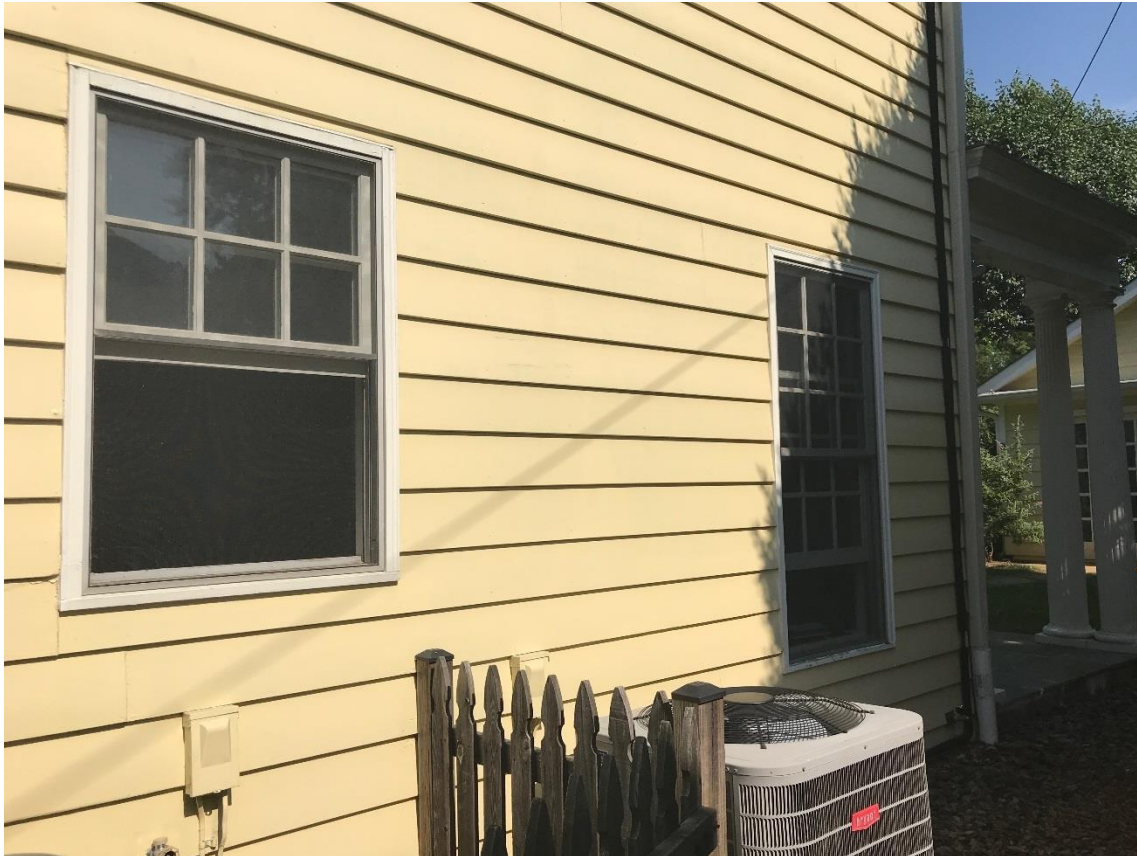
Figure 2: The replacement (right) window will match the shorter existing kitchen window (left).
