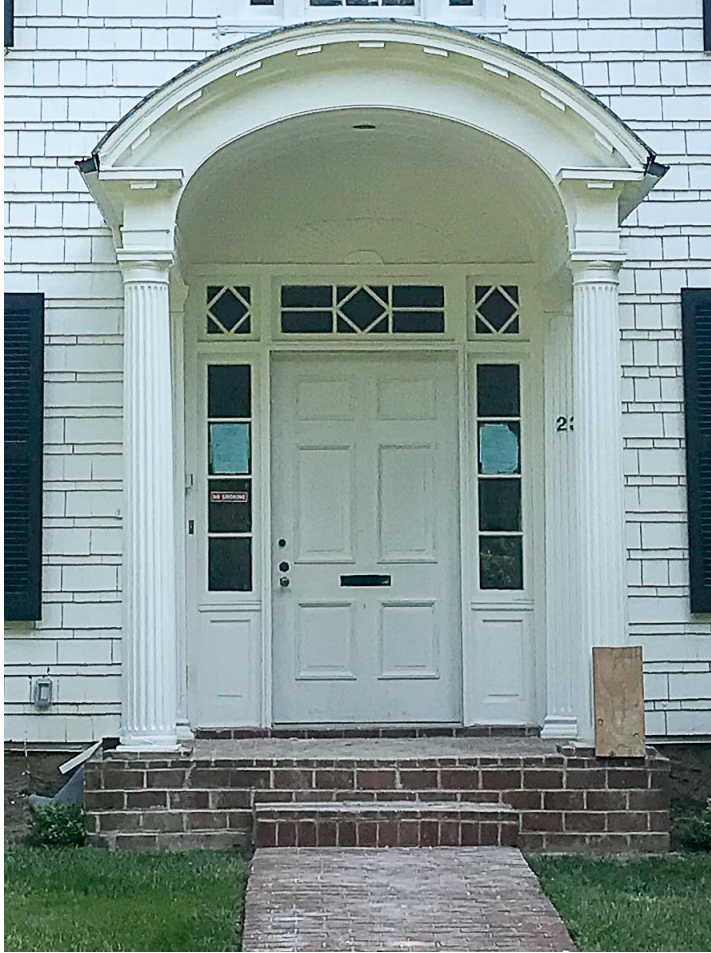
Figure 4: the front porch brick cladding and steps are non-historic alterations.
