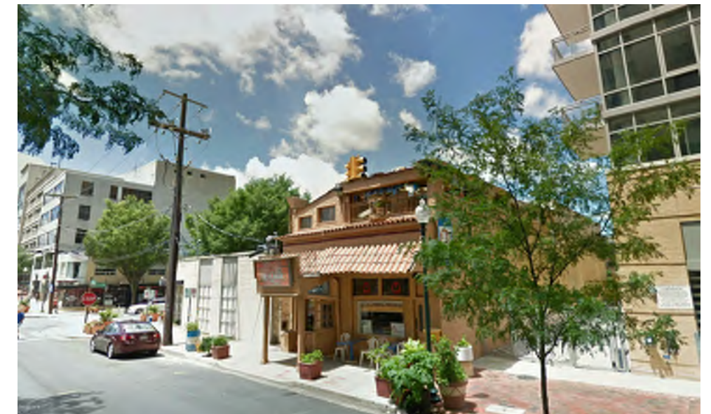
6. DEL RAY AVE LOOKING SOUTHWEST
