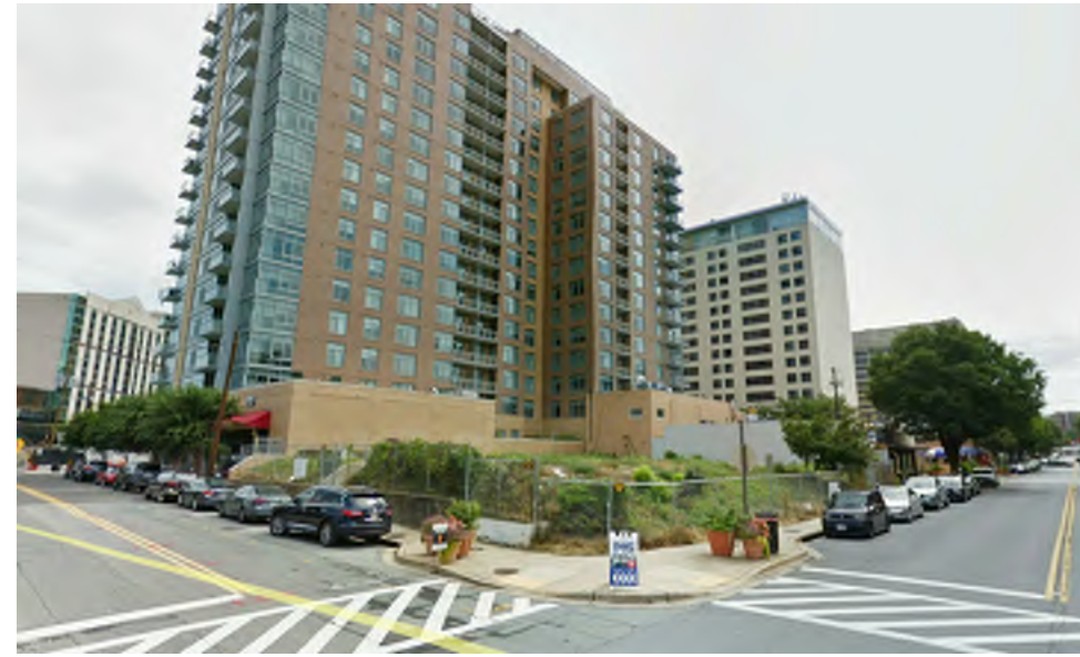
2. CORNER OF AUBURN AVE AND NORFOLK AVE
