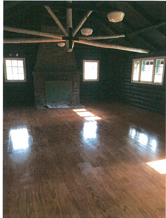
Interior view of windows
