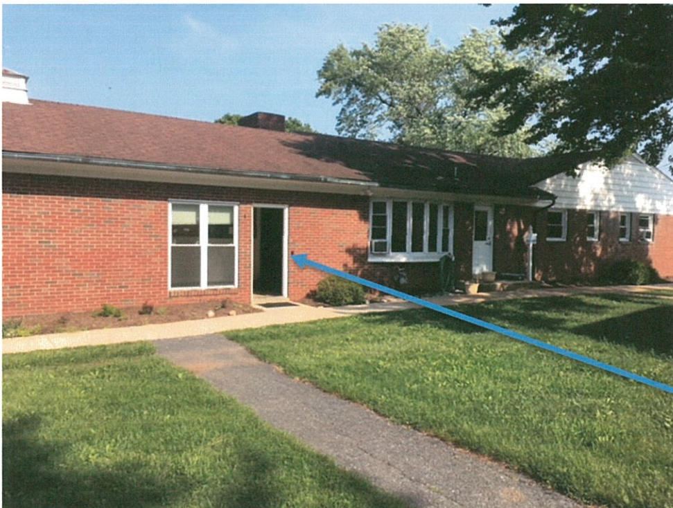
West side of the Manse with door entrance location for the handicap ramp. The window next to the door will be replaced with a shorter window to accommodate the ramp being attached alongside the building.
