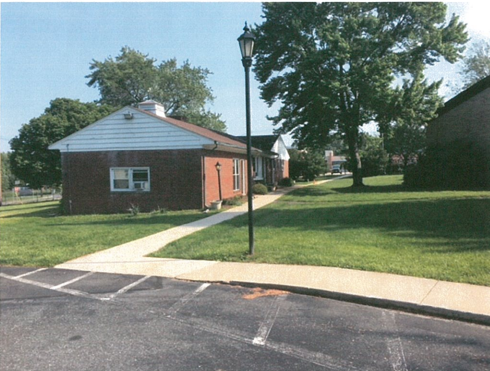
North side of the Manse showing path of access from the parking lot via sidewalk.
