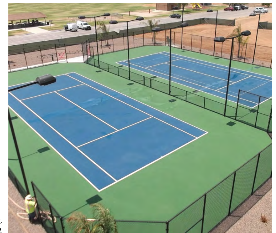
Public tennis courts, Miramar, FL
