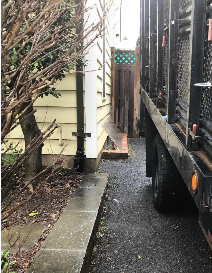
Figure 3: Window well from further down the driveway.
