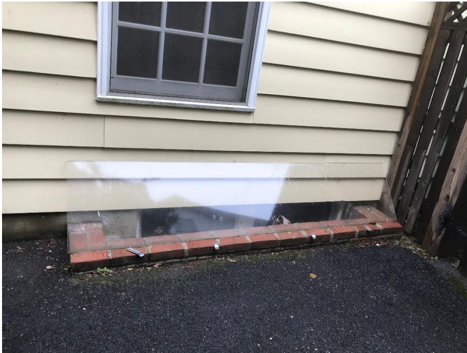
Figure 2: Photo of existing window well.
