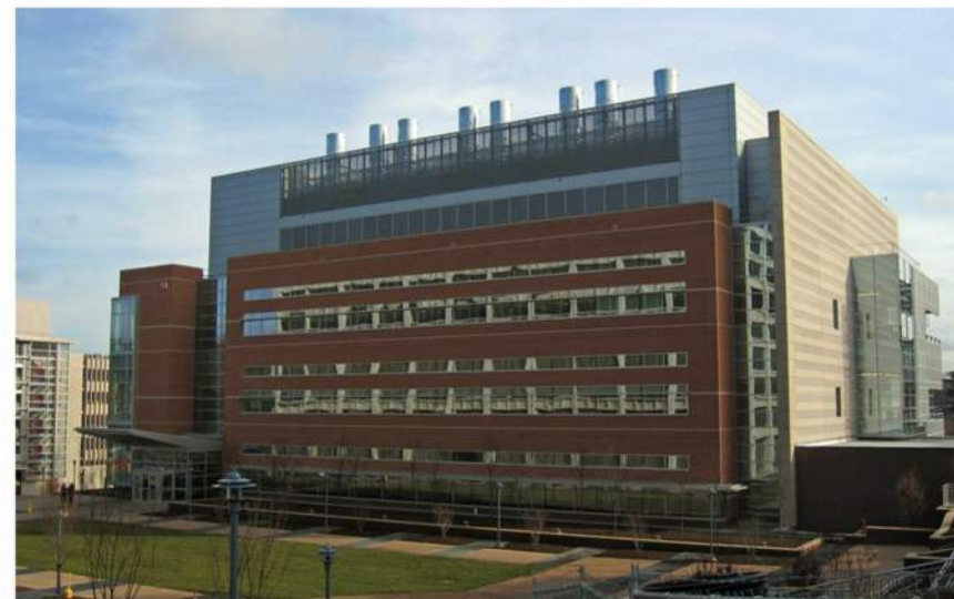
NIH BUILDING 33 BETHESDA, MARYLAND
