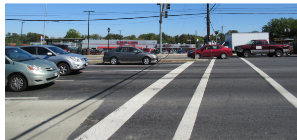
Example of a long pedestrian crossing with no median refuge island at Randolph Road
