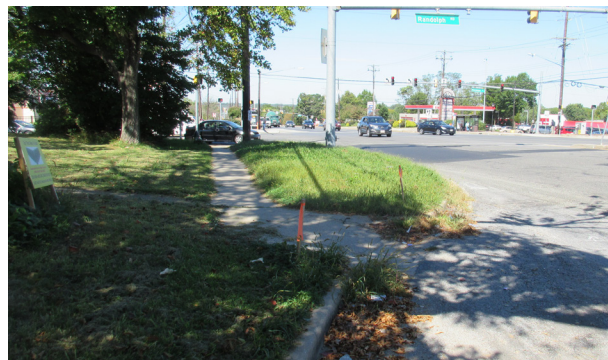
ADA non-compliant ramp
