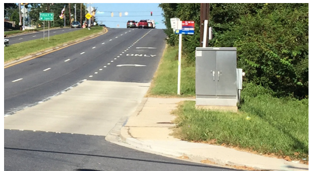
Continuous turn lane and no sidewalk connection to bus stop
