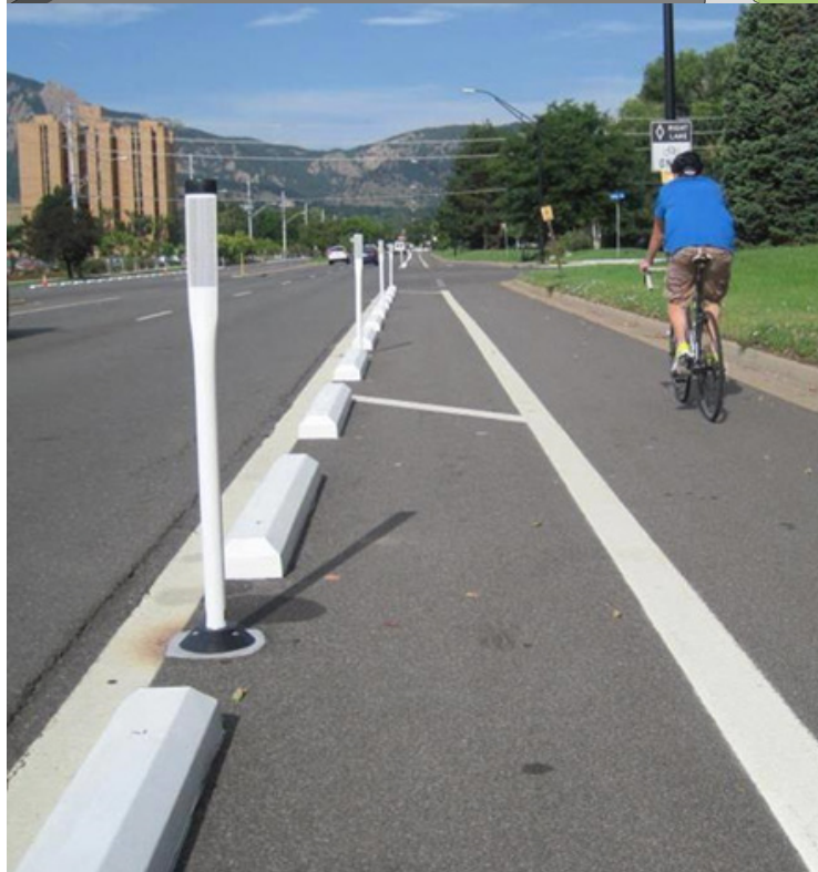
Cost-efficient rapid-implementation variation of a two way separated bike lane on Baseline Road in Boulder, CO.
