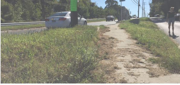
Sidewalk blocked with mowing debris
