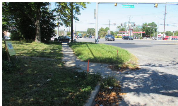
ADA non-compliant ramp
