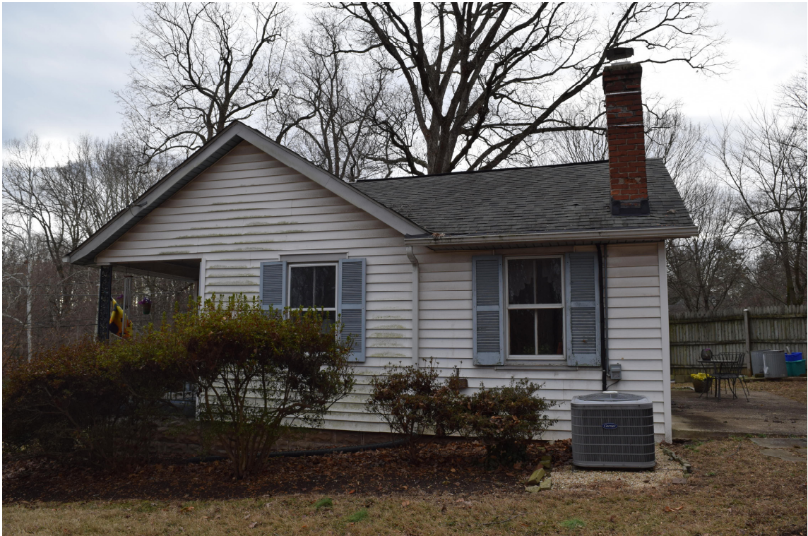
b. Existing Right Side of 4601 Waverly Avenue
