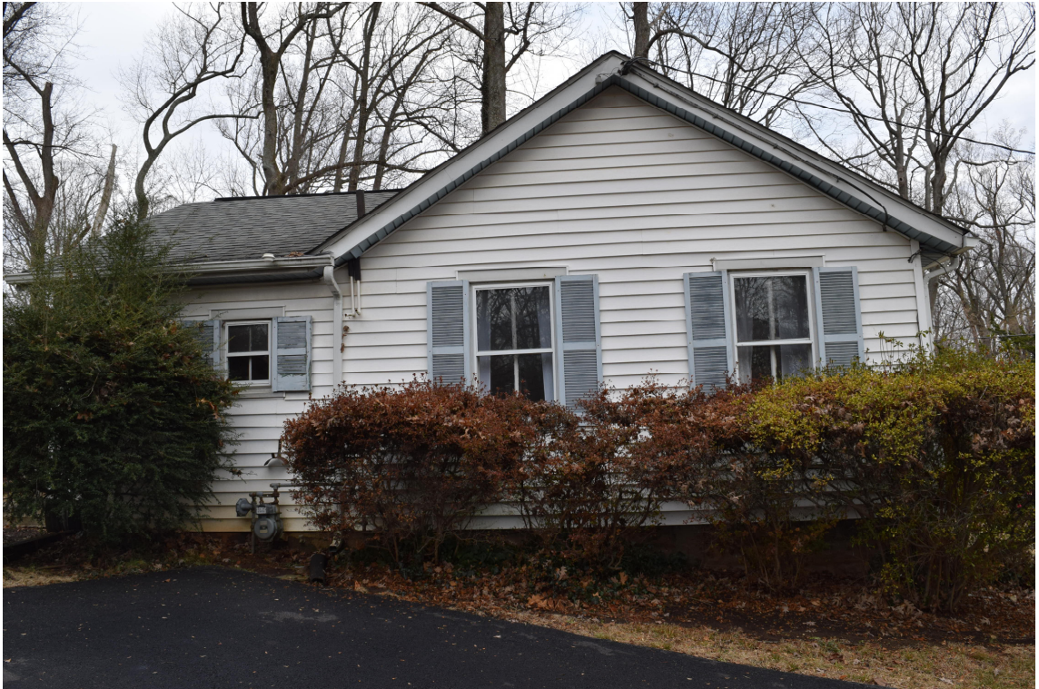
d. Existing Left Side of 4601 Waverly Avenue
