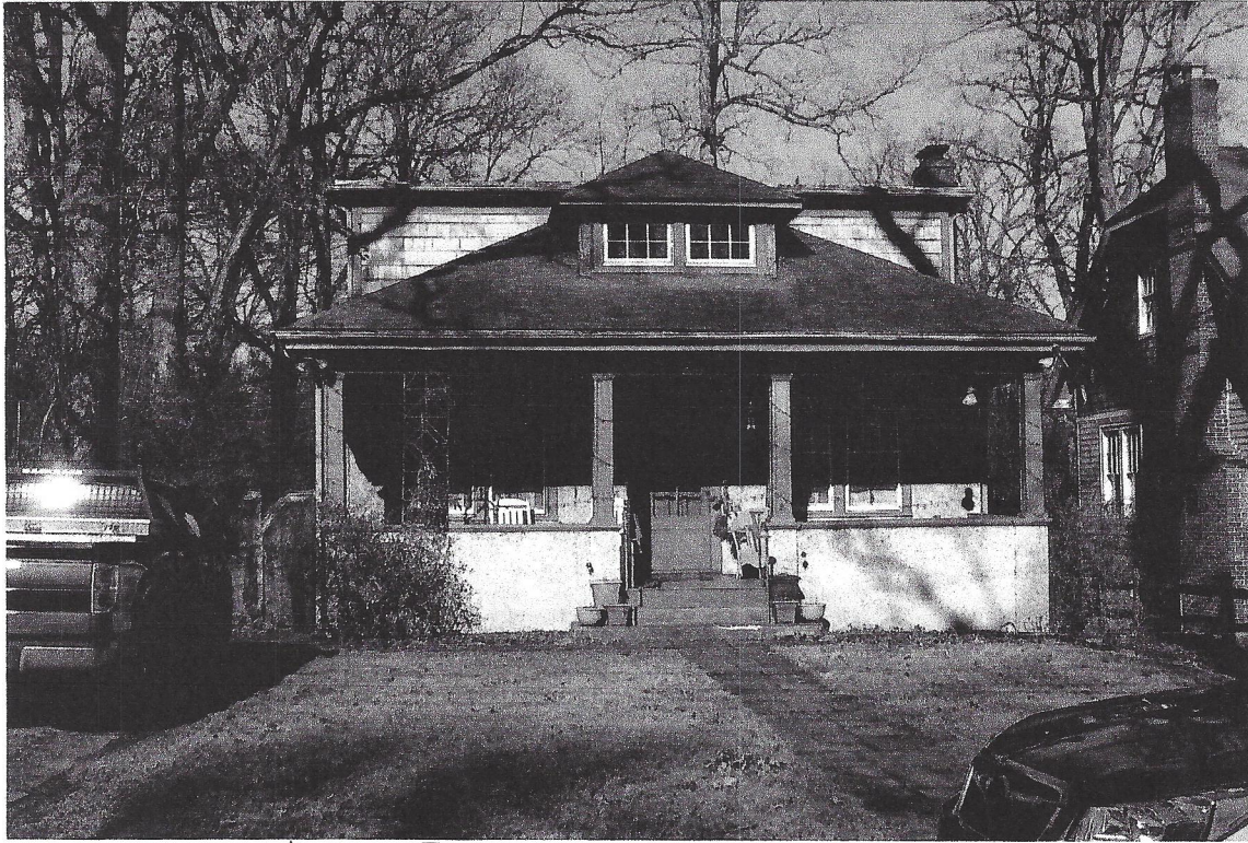
Detail: SOUTH FACADE
