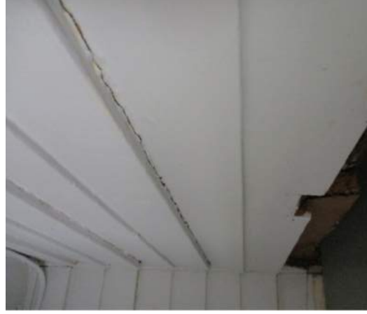
ORIGINAL HOUSE SIDING
