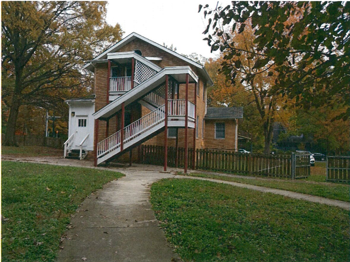
Rear View - Existing
