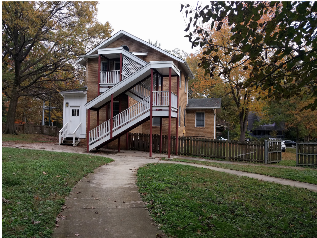
Rear View- Existing
