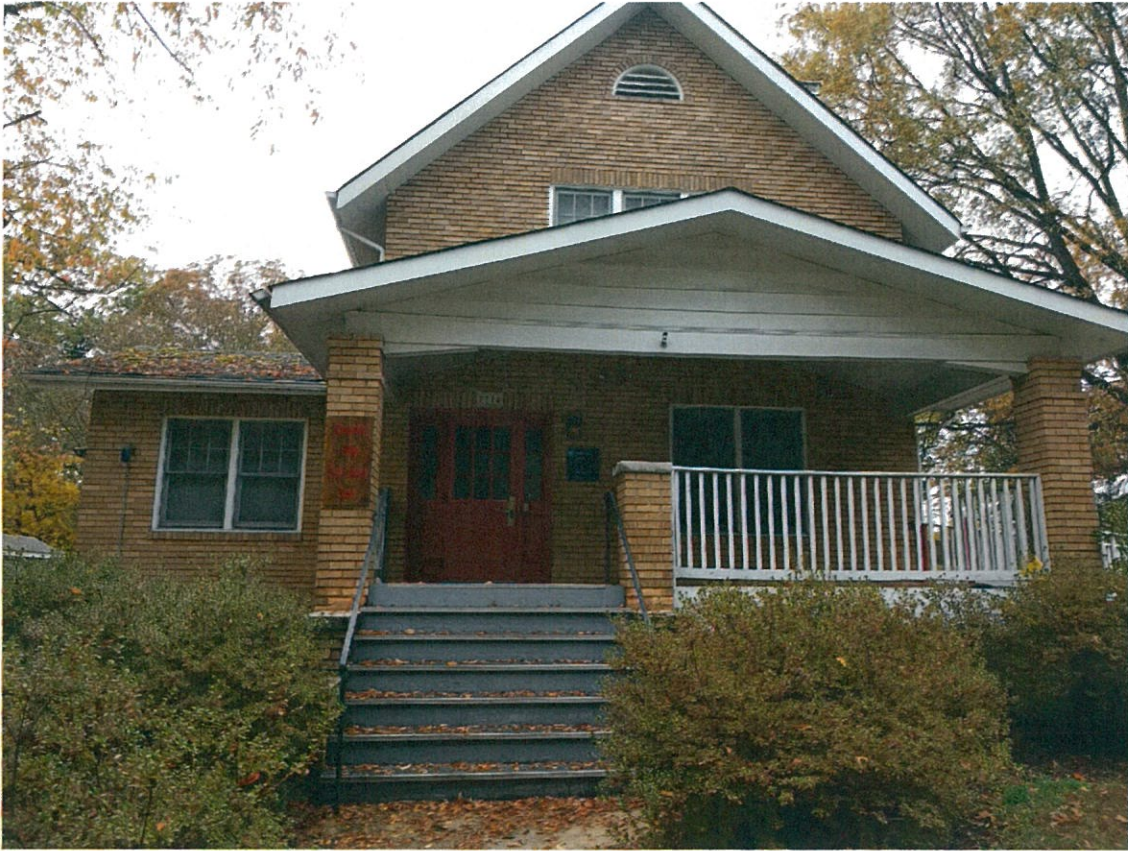
Front View - Existing
