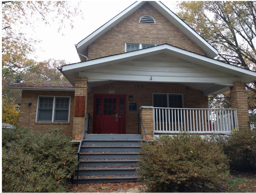
Front View- Existing
