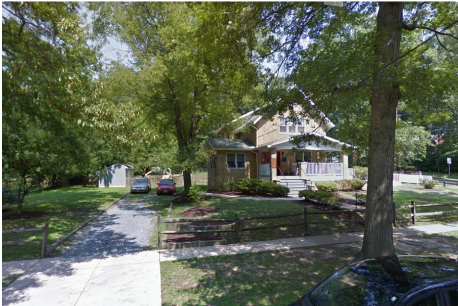
Figure 1: View from Takoma Ave toward proposed addition
